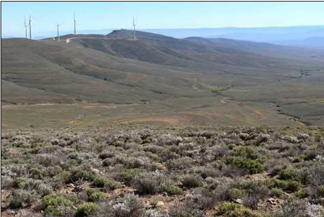
Figure 5: View from the Brakeinde ridge into next valley to the north, Ekkraal 199. Bedrocks are exposed along deeper stream gullies but these will be spanned by the proposed 132 kV powerline. Anticipated impacts along drainage lines will be mainly attributable to any associated new access roads.
