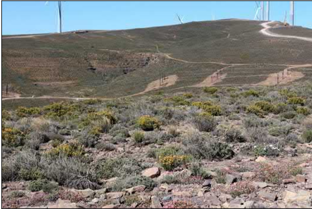
Figure 8: New wind farm infrastructure on Ekkraal 199, some 2 km west of the new Eskom substation on Bon Espirance 93, showing the substantial area of surface disturbance associated with even small-scale overhead powerlines (middle ground). Sectors of wind turbine access road also require the excavation of major new road cuttings into Abrahamskraal Formation bedrocks.
