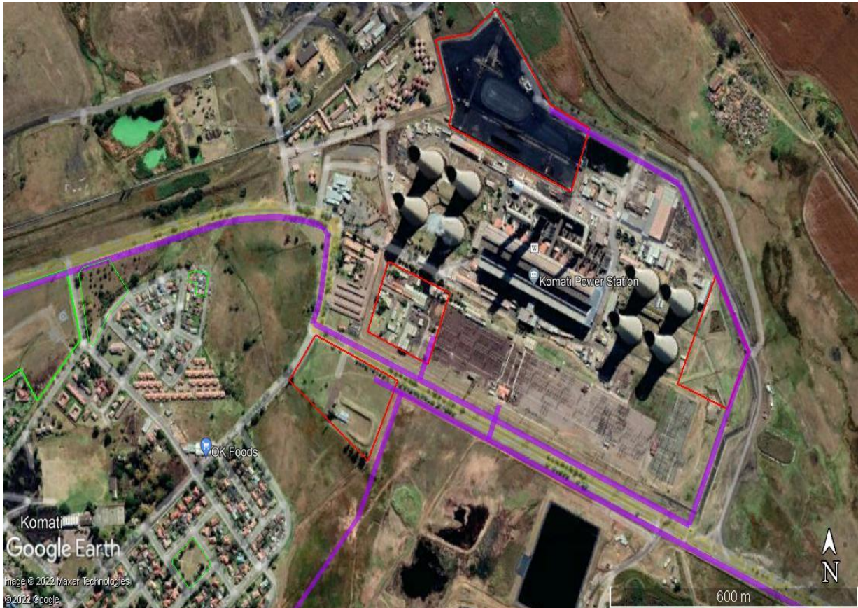
Figure 5: Closer view of the Komati Power Station area with sections of the powerlines in purple and the BESS areas in red shown. The heavily disturbed nature of the area is clear (Google Earth 2022).
