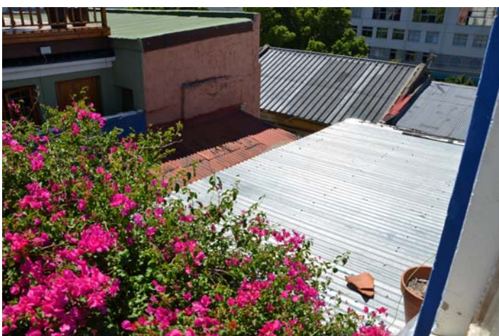
Courtyard & building seen from first floor
