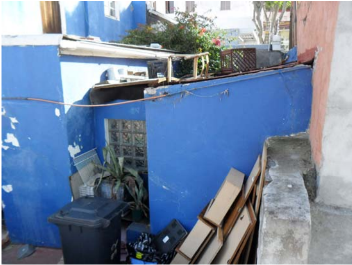
Out house connected to rear of building
