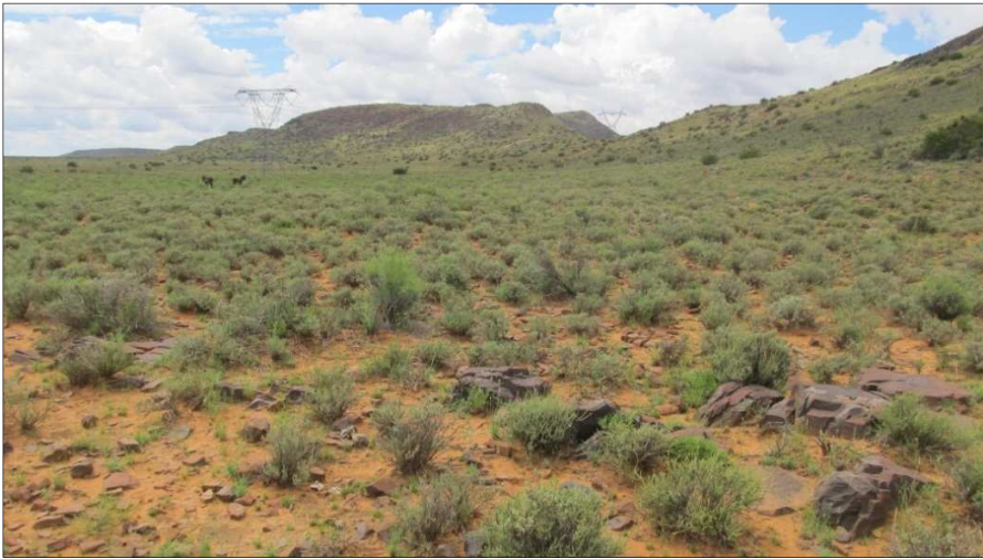
Figure 4. Construction Yard 1 view facing north east
