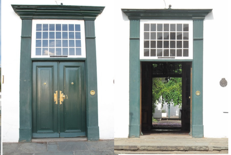
Front door detail [east elevation]
