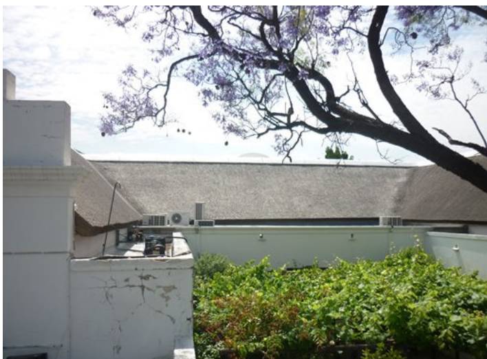
Roof structure [facing east]
