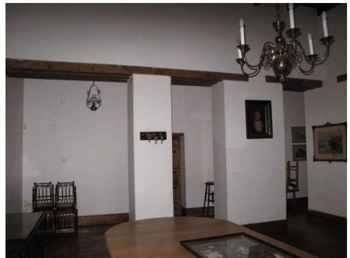
Wijnkamer [looking north towards passage and access door to courtyard]
