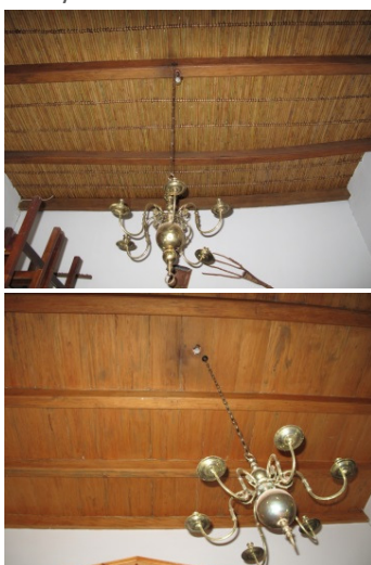
Ladies bar ceiling detail [reed in hearth room]
