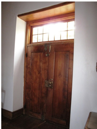
Lounge door to courtyard detail
