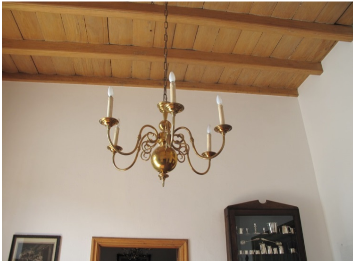
Typical ceiling and light fitting detail [entrance foyer to dining hall]
