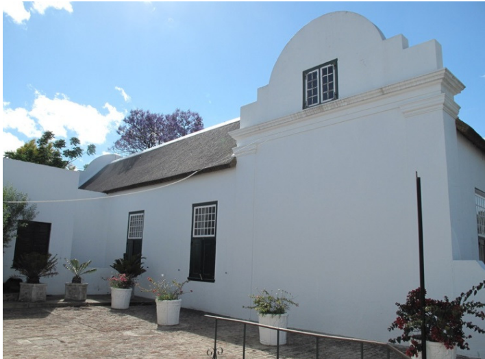
South elevation [dining hall internal & Camdeboo courtyard]
