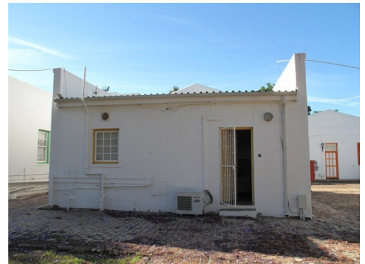
Back (south) facade
