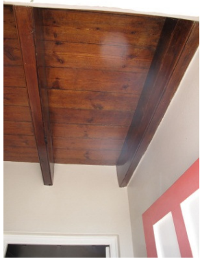
Oregon foyer and bedroom A ceiling; bedroom B floor (carpeted)
