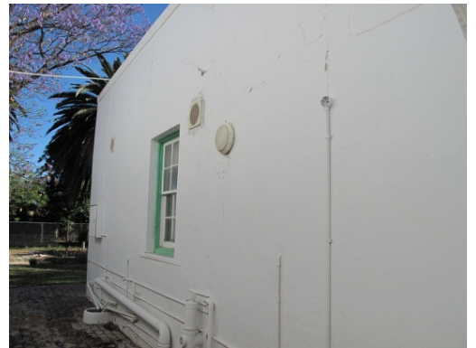
Side (east) facade
