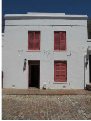
Front (north) facade
