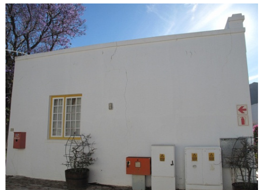
Side (east) facade
