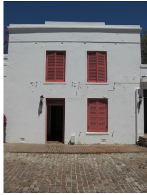
Front (north) facade
