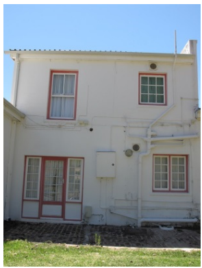
Back (south) facade
