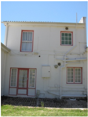
Back (south) facade
