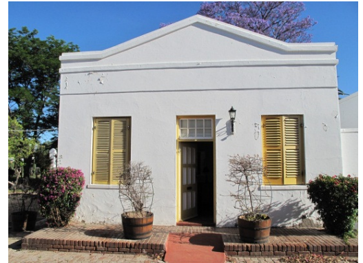
Front (north) facade
