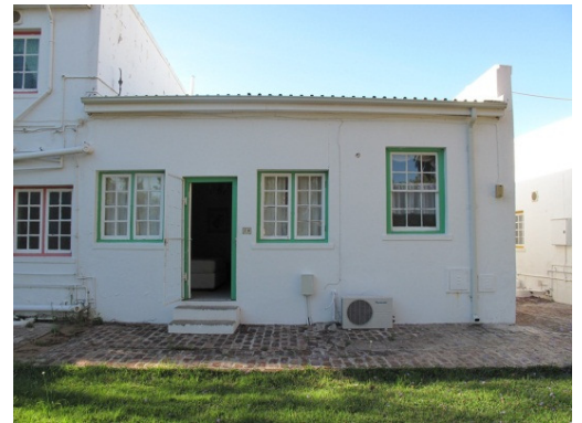
Back (south) facade
