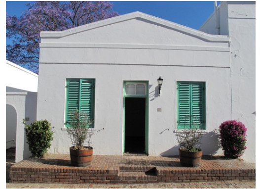
Front (north) facade
