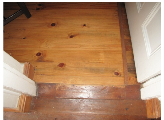
Bedroom B & C: Pine wood strip floor (patched in part)
