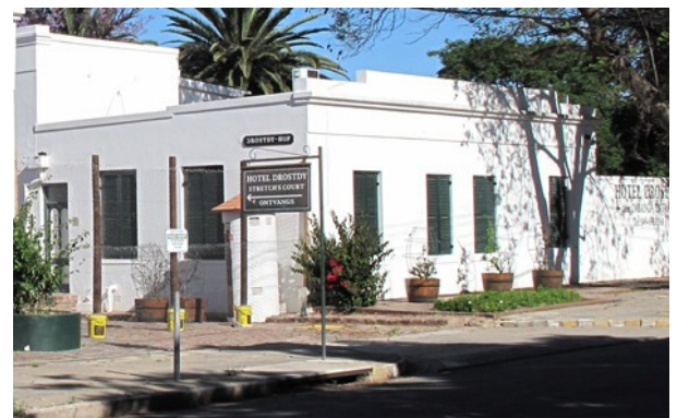
Side (west) façade on Bourke Street
