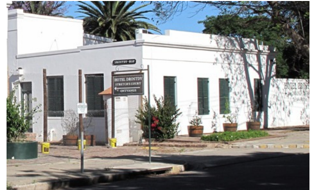
Side (west) façade on Bourke Street
