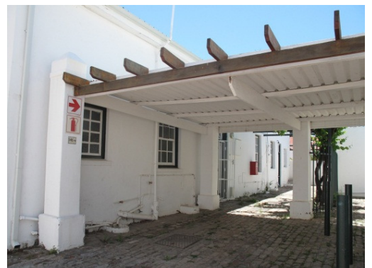
Back (east) façade to room C
