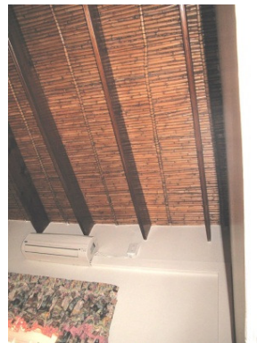
Bedroom A: Oregon beams and reed ceiling
