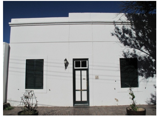
Front (west) façade to rooms D & E
