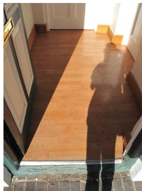
Foyer D & E: laminate floor
