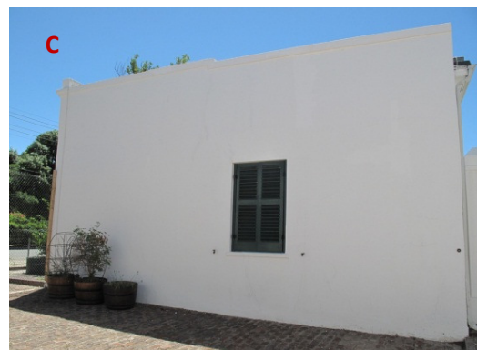
Side (south) facade
