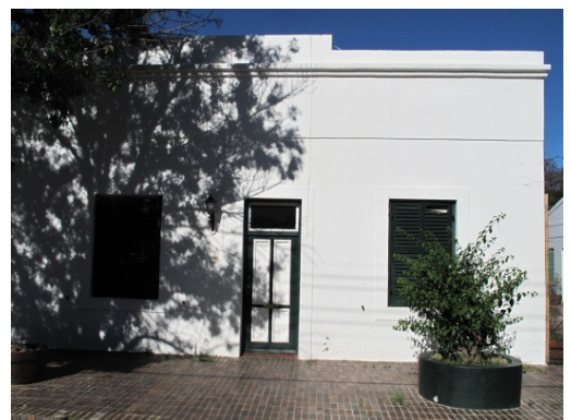
Front (west) façade to rooms A & B
