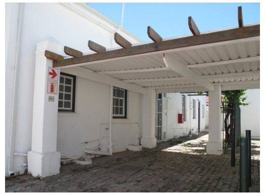
Back (east) façade to room C
