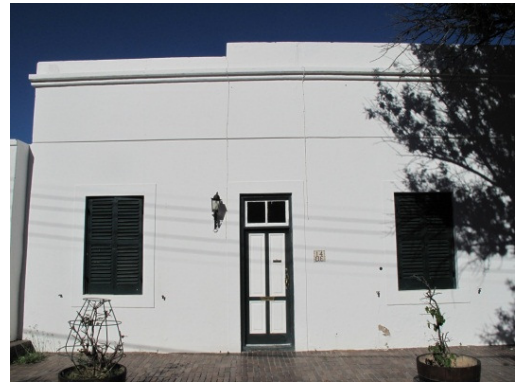
Front (west) façade to rooms D & E
