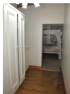
Bedroom A passage: Oregon Pine ceiling and floor
