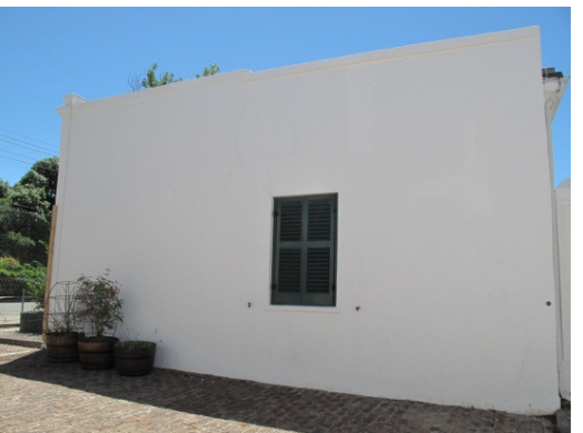
Side (south) facade
