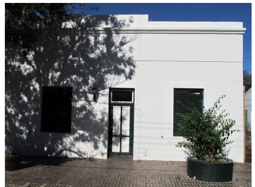
Front (west) façade to rooms A & B
