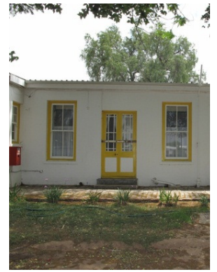
Back (south) facade
