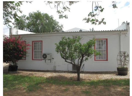
Back (south) facade
