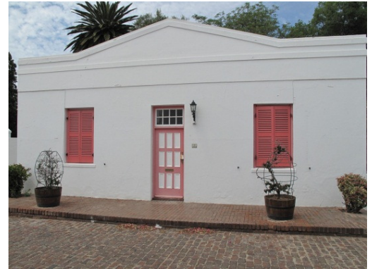
Front (north) facade
