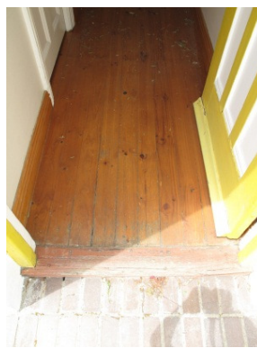
Foyer / passage: Oregon Pine wood strip floor
