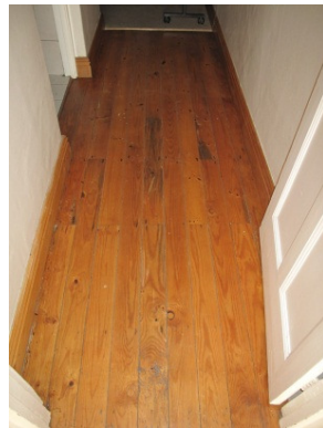
Bedroom A: Oregon Pine wood strip, and carpeted concrete floor
