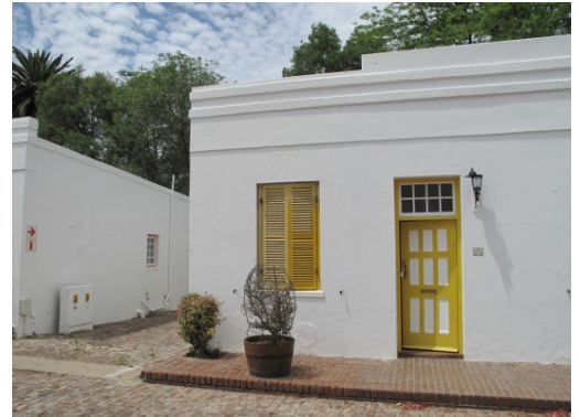
Front (north) facade
