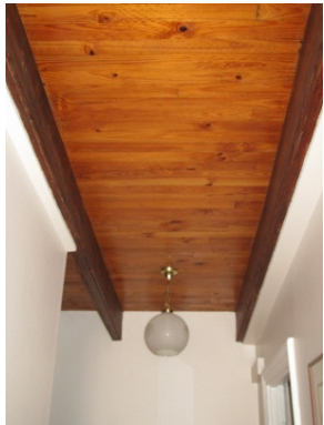
Back passage: Oregon Pine ceiling and beams
