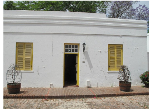
Front (north) facade
