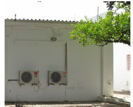
Back (south) facade
