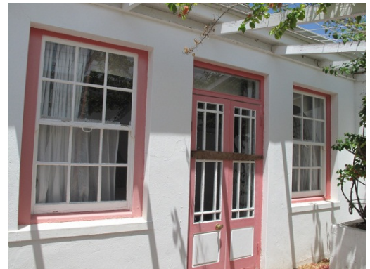
Back (north) facade
