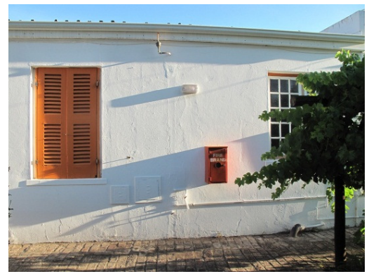
Back (north) facade
