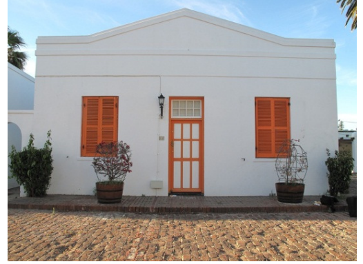
Front (south) facade
