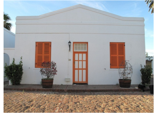
Front (south) facade
