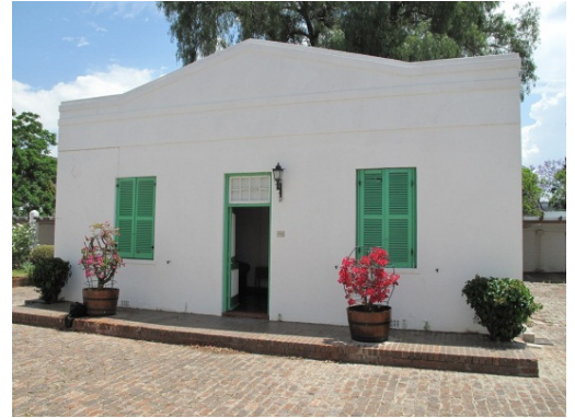
Front (south) facade
