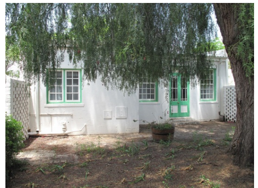
Back (north) facade
