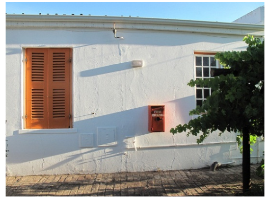
Back (north) facade
