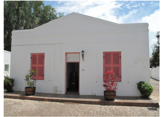
Front (south) facade
