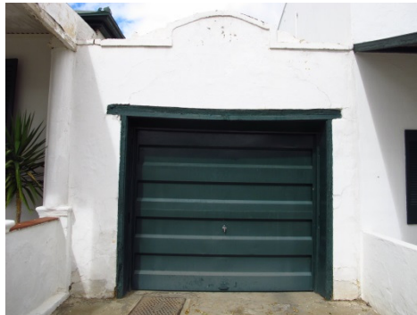
Garage / coach house entrance with aged timber lintel
