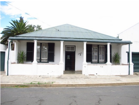
No 5 Parlement facade
