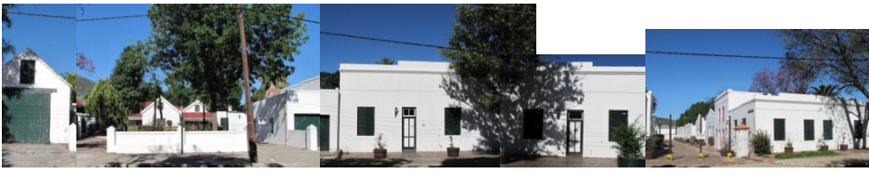
3. Bourke Streetscape (from left to right – Ferreira House, no's 14 and 15)
