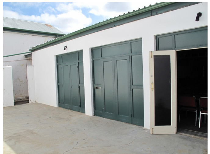
Thibault Room rear extension façade [west elevation]
