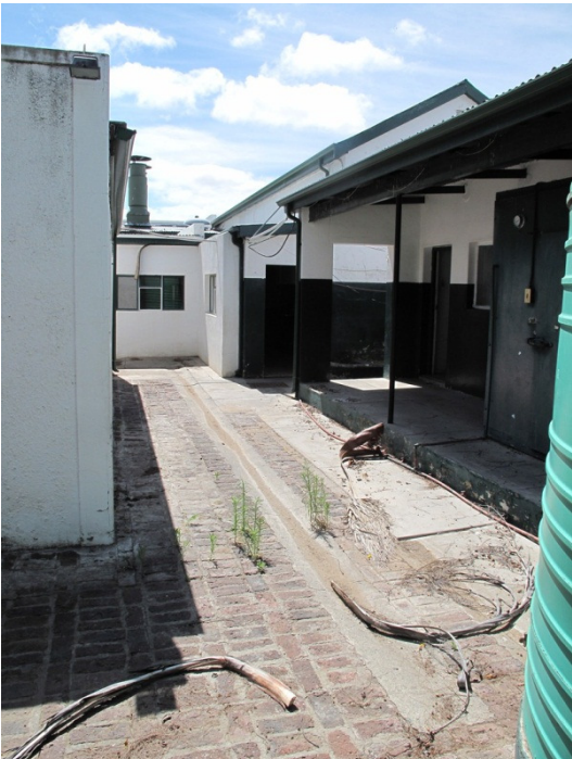
Drostdy kitchen Back of House and stores [south wing]
