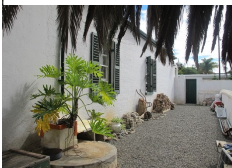
East façade adjacent to Kromm's Inn
