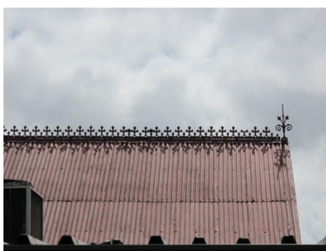
Thibault Room ridge line with cresting
