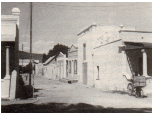
FIGURE 31: Stretch's Court before restoration c. 1968 [Mark Senekal]
