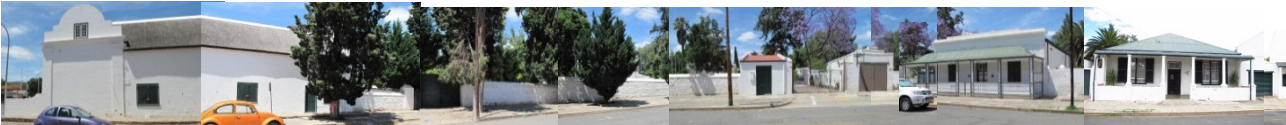
2. Parlement Streetscape (from left to right – Drostdy, historic wall, Cobbler's Shop, Kromm's Inn, No. 5 Parlement Str)
