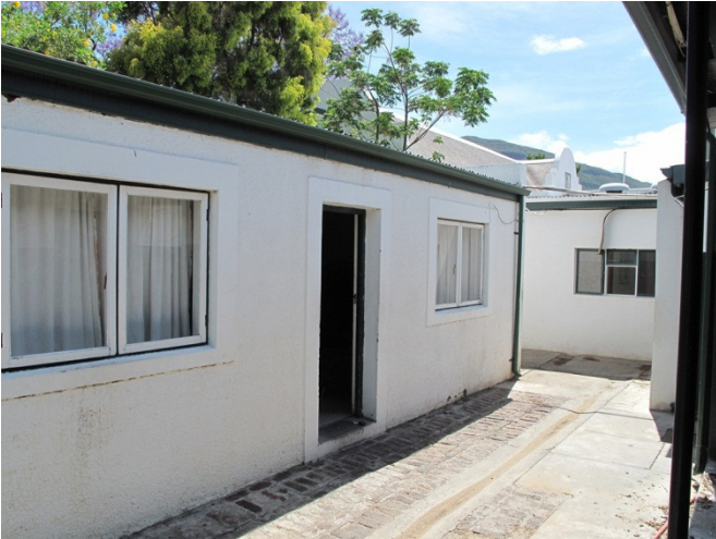
Drostdy kitchen Back of House and stores [south wing]
