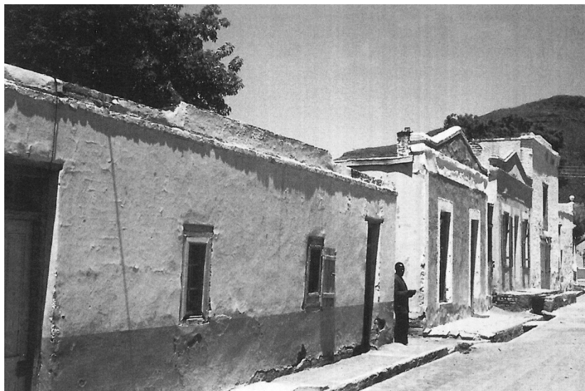
FIGURE 34: Stretch's Court from left to right c. 1965, prior to restoration – no 4 with west addition, no's 3, 2, 1 and 15 on the corner [Fransen 2006]
