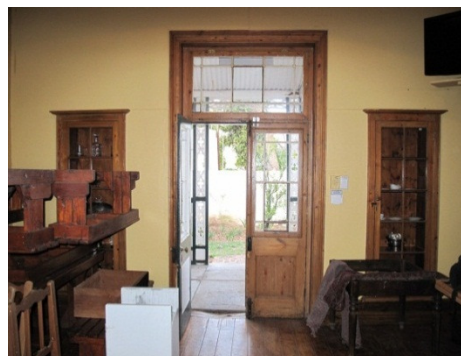
East elevation access door
