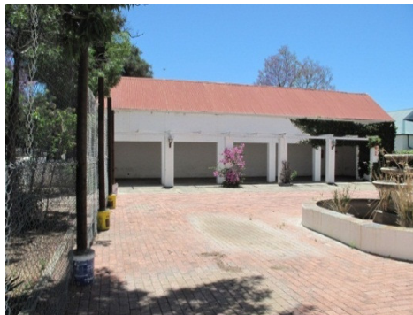
Ferreira House garage south elevation
