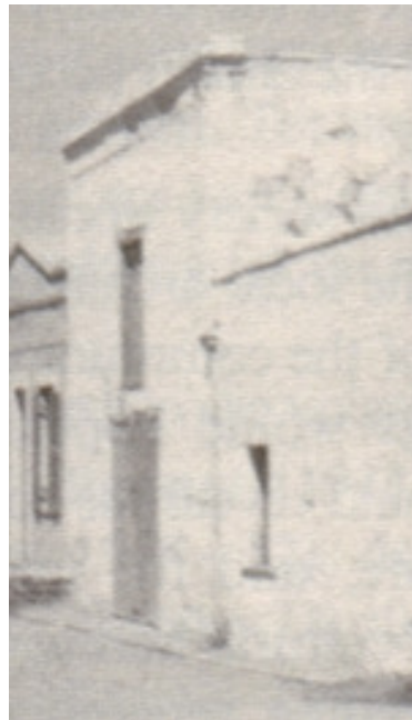
No. 1 Stretch's Court prior to restoration [Mark Senekal]
