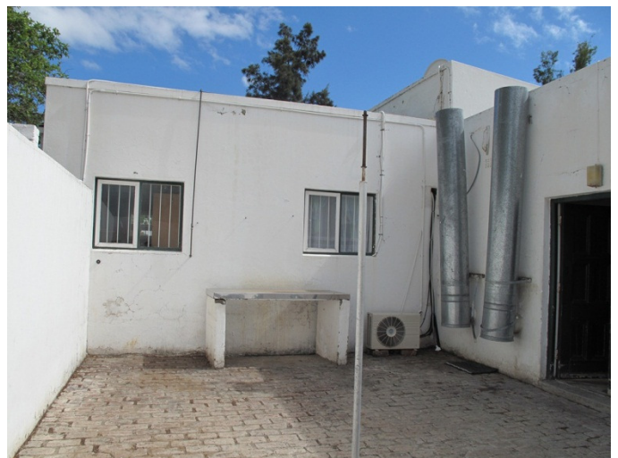
Laundry room and housekeeping store
