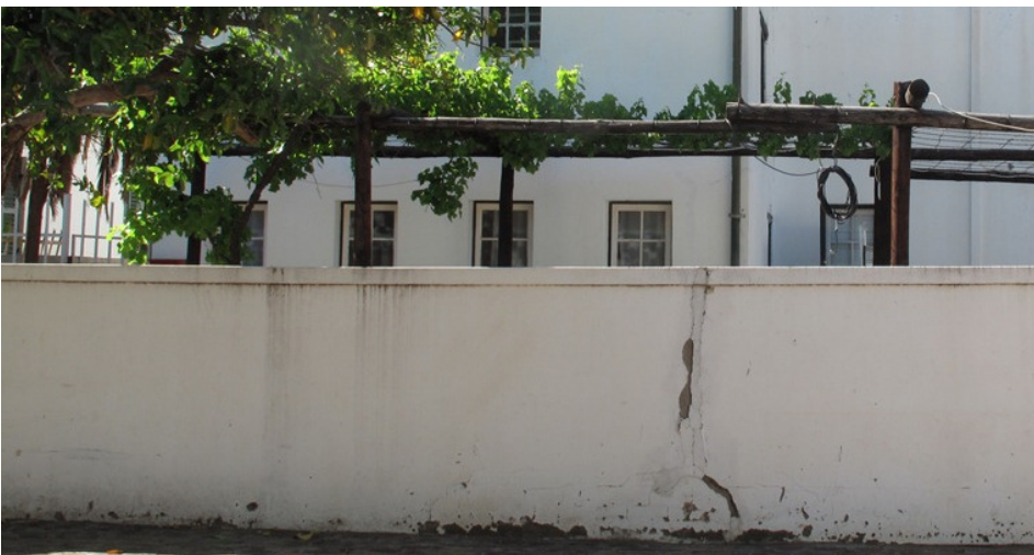
Wall dividing Kromm's Inn and the additional parking court
