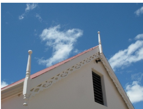
Ferreira House gable trim
