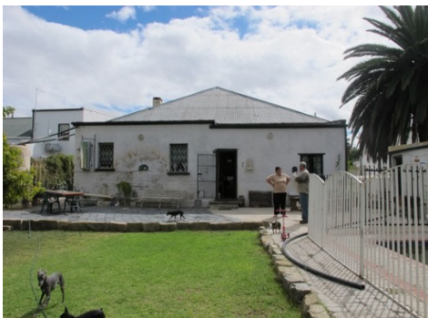
South (rear) façade of later lean-to addition
