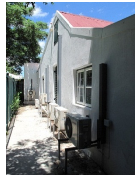
East elevation roofline
