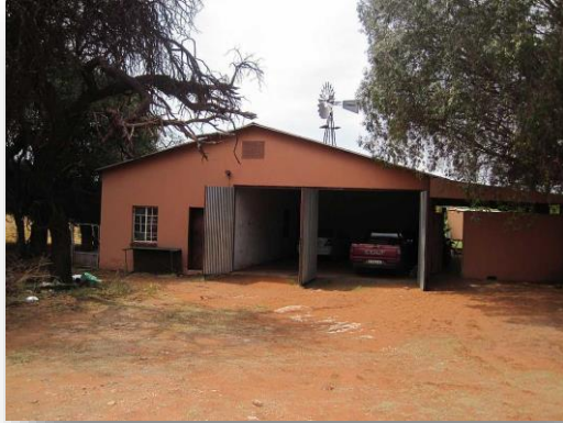
Figure 29: Stone shed at site K13
