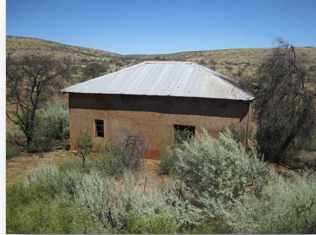
Figure 26: Walling of stock enclosure at site K7
