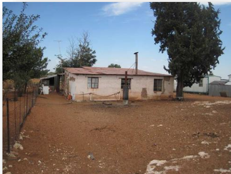
Figure 29: Stone shed at site K14
