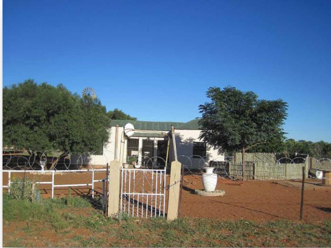
Figure 25: Ruined house at site K2
