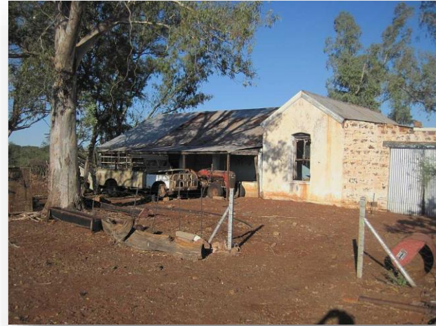
Figure 29: Stone shed at site K15
