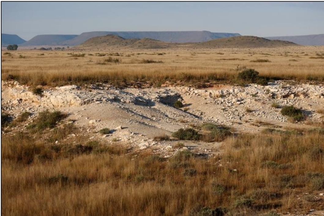
Figure 23: Good borrow pit exposure of the pervasive, thick calccrete hardpan overlying most of the low-lying terrain within the Kudu renewable energy project area, seen here on farm RE/197, outside and c. 4.7 km west of the project area itself.
