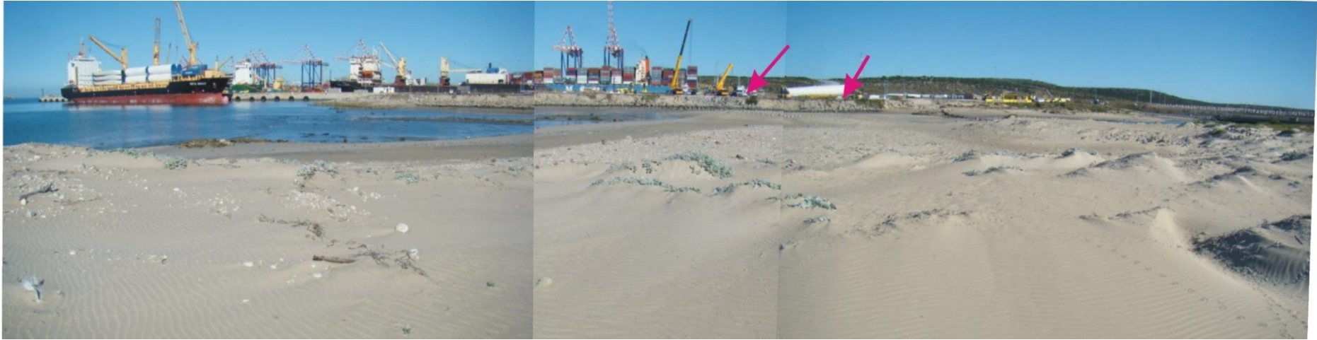
Figure 12.11. The harbour, looking southwest. The area allocated for the construction of the proposed General Cargo Berth (B101) is underlain by reworked bulk sediments used to construct the existing harbour quay (arrows).
