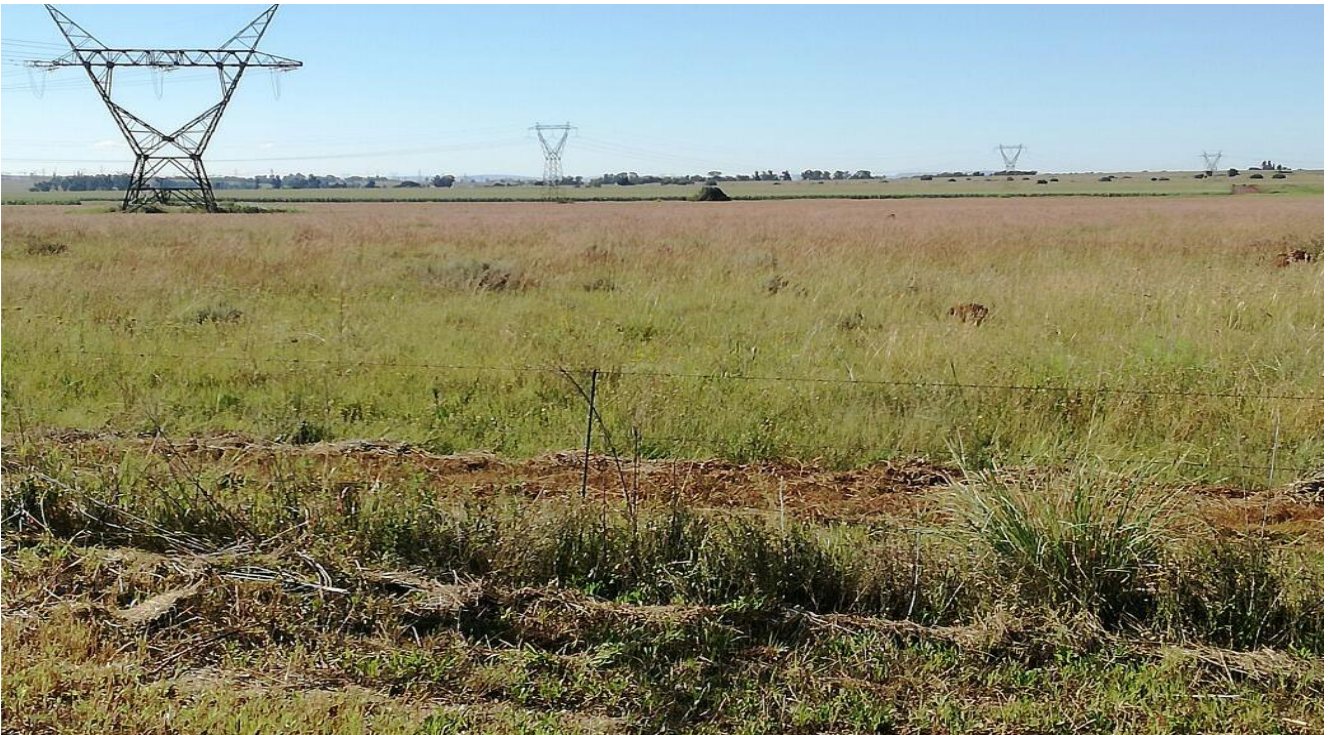
Plate 8: Photo 8: View of existing powerline from Pluto substation to Watershed substation (Photograph © by Author 2018). Note that the proposed Alternative 2a route will run parallel to the existing 275kv line
