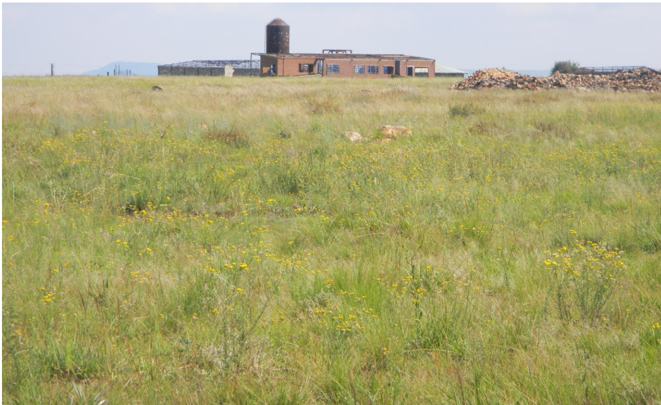
Plate 25: Photo 25: View of abandoned farm buildings and mine diggings on the Farm Wildfontein along Alternative 2a powerline route (Photograph © by Author 2018)
