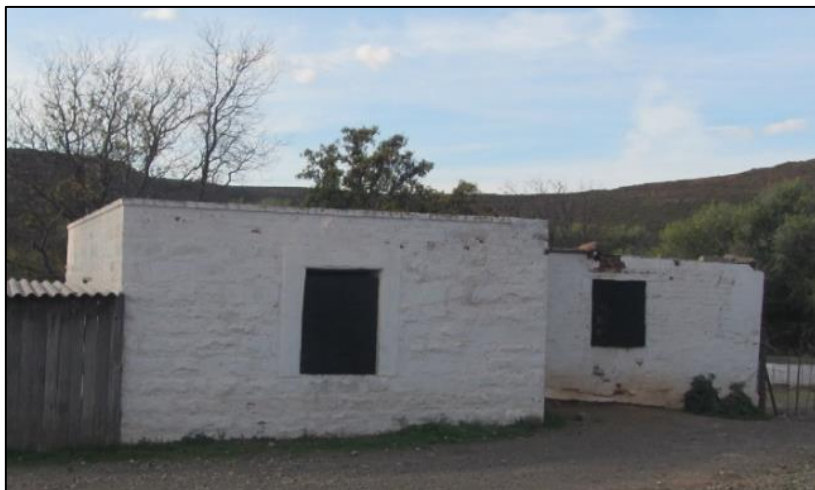
Figure 31: Structure in the Leeukloof Farm complex at Waypoint 1850. Source: Orton (2021a: fig. 50).
