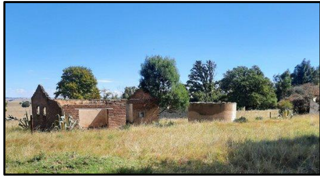
Figure 8.3. additional buildings at CA001.
