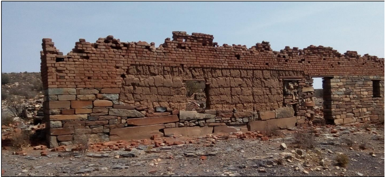
Figure 37: A structure built of stone, sun-dried mud bricks and fired clay bricks at Waypoint 1993. Source: Orton (2021a: fig. 30).
