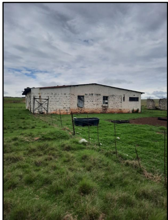
Figure 8.9. Structure at DN073
