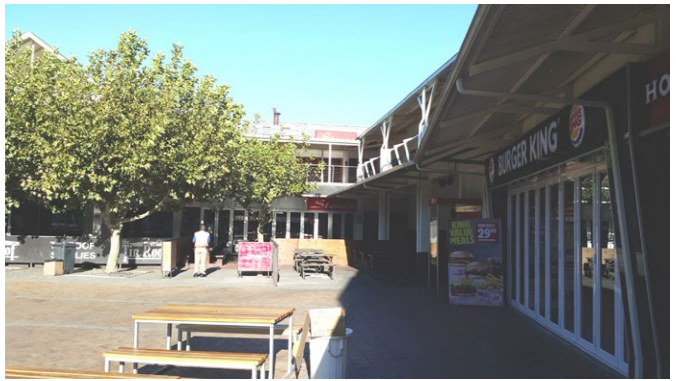
EXISTING BUILDINGS TO BE DEMOLISHED
