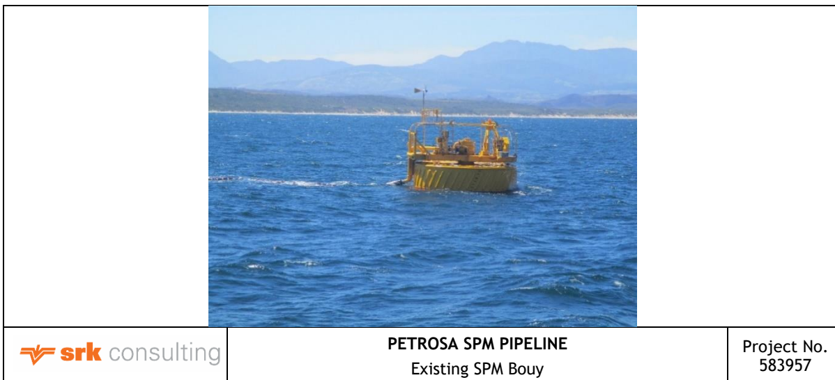
Figure 1-2: Existing SPM buoy
