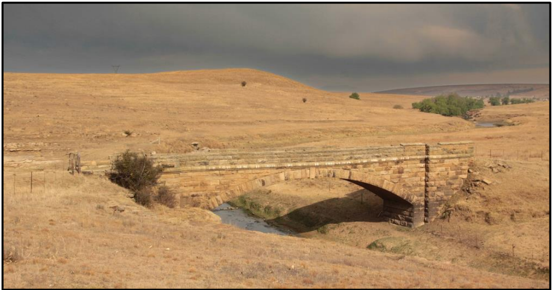
Figure 8. Swalu bridge near Harrismith
