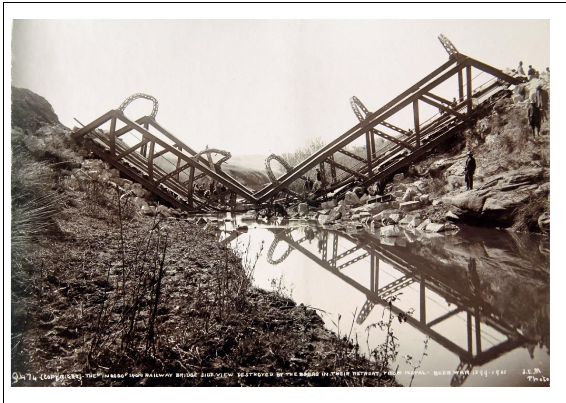
Figure 11. The railway bridge across the Ngogo River, destroyed by the retreating Republican forces (Image: Private collection)
