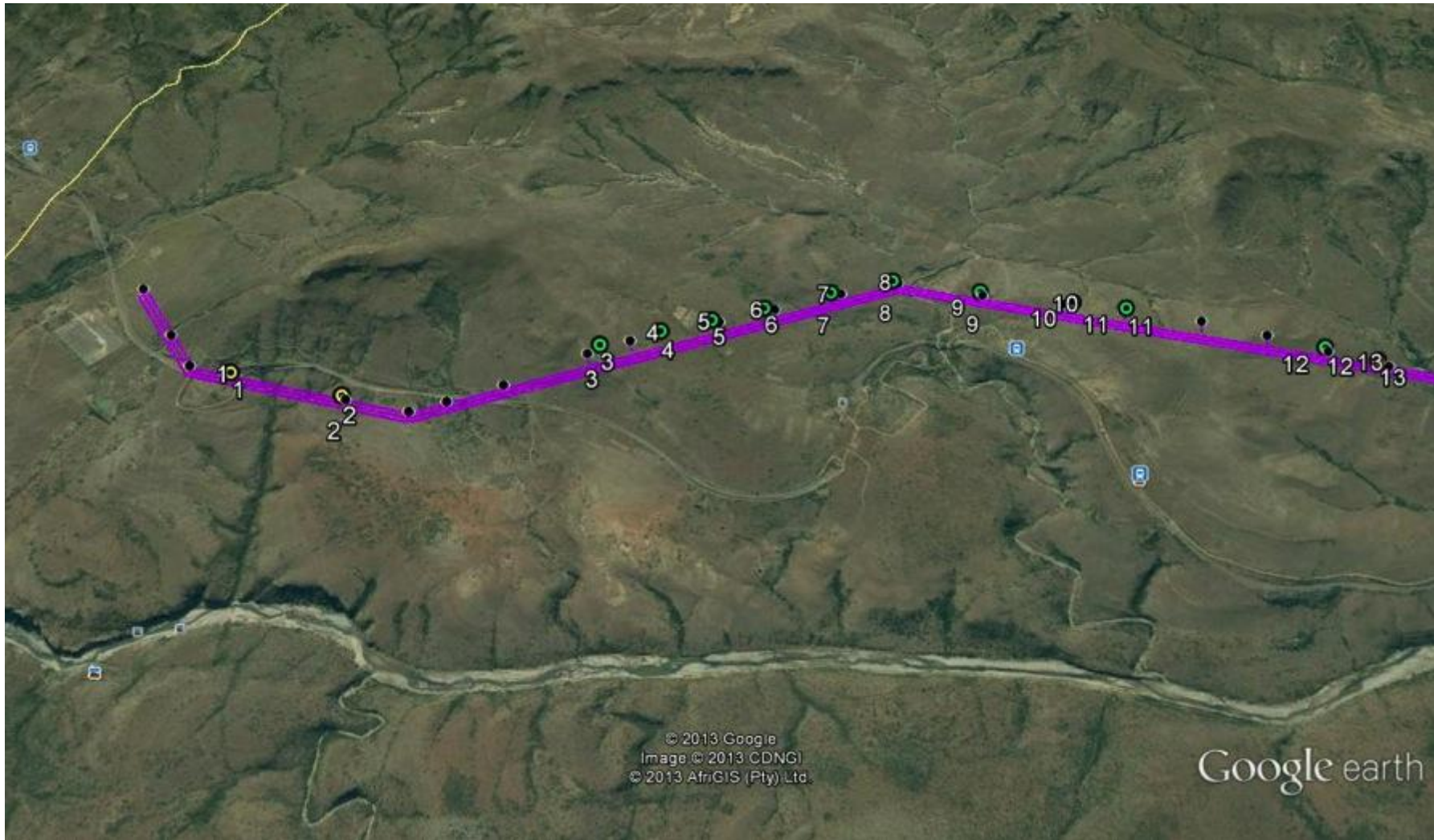
Figure 2: The powerline pylon positions follow the servitude that runs parallel to an existing high voltage powerline and railway line.
