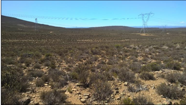
Figure 7: View of the area proposed for substation alternative SS1 facing north (Fortuin 74).
