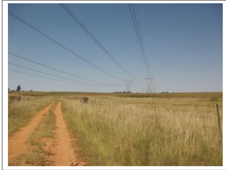
Figure 4- Dirt roads here and there criss-cross the project area and assisted with the survey of the road alternatives. Alternative F runs along Eskom's existing 400kV power lines (above).
