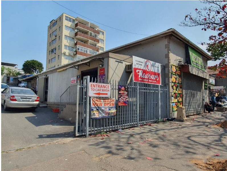
A prefab building has been added to the east side of the shop
