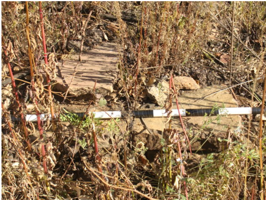
Figure 23: Remains of a building at site no. 1.
