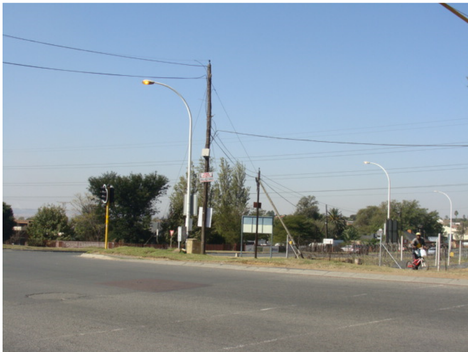
Figure 13: Intersection at OR Tambo Road where the proposed extension will start.
