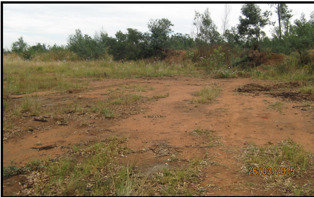
Figure 13: An embankment of the above area shows the shallow yellow sandstone.
