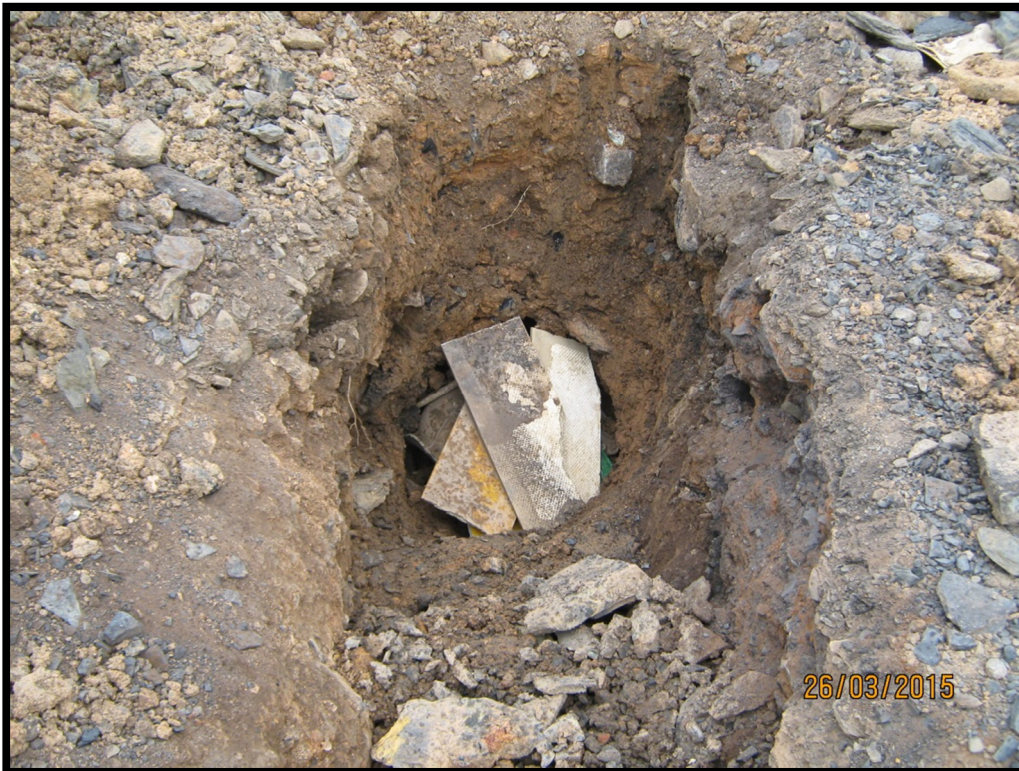
Figure 8: A trench dug to expose services, the darker grey represents the shale and the yellow represents the sandstone. No formal layering was observed. The rocks on the surface are from previous mining activities.
