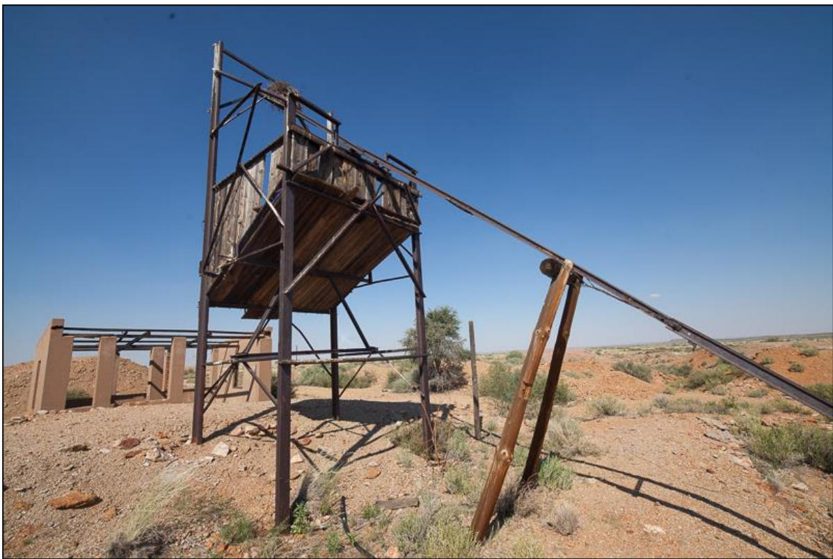
Figure 14 -- Headgear at the abandoned tungsten mine on Portion 12 of Dyason's Klip 456. The mine area (about 3,5 ha) will require mitigation should development encroach closer than 50 m.
