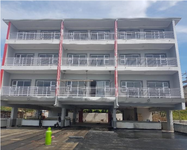
Plate 5: Ground Level, Parking Deck.
