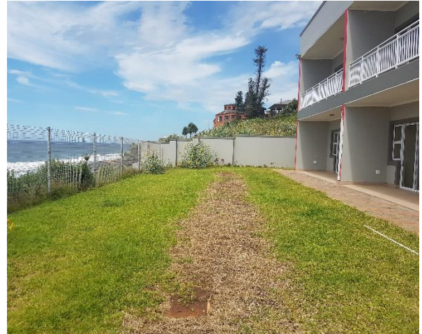
Plate 2: Basement Level View.
