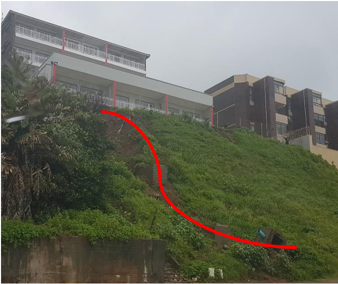
Plate 9: View of the Bank on Seaward Side of the Property.
