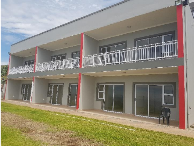
Plate 1: Apartments at Basement Level, Sea View.
