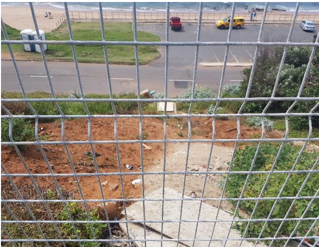
Plate 3: View of the Bank on Seaward Side of the Property.
