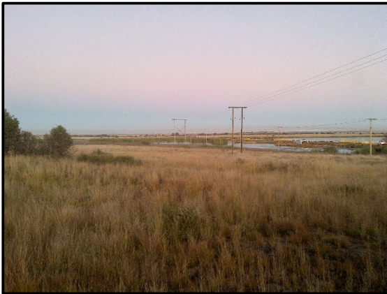
Figure 5: Existing powerline in the southern section of the study area.
