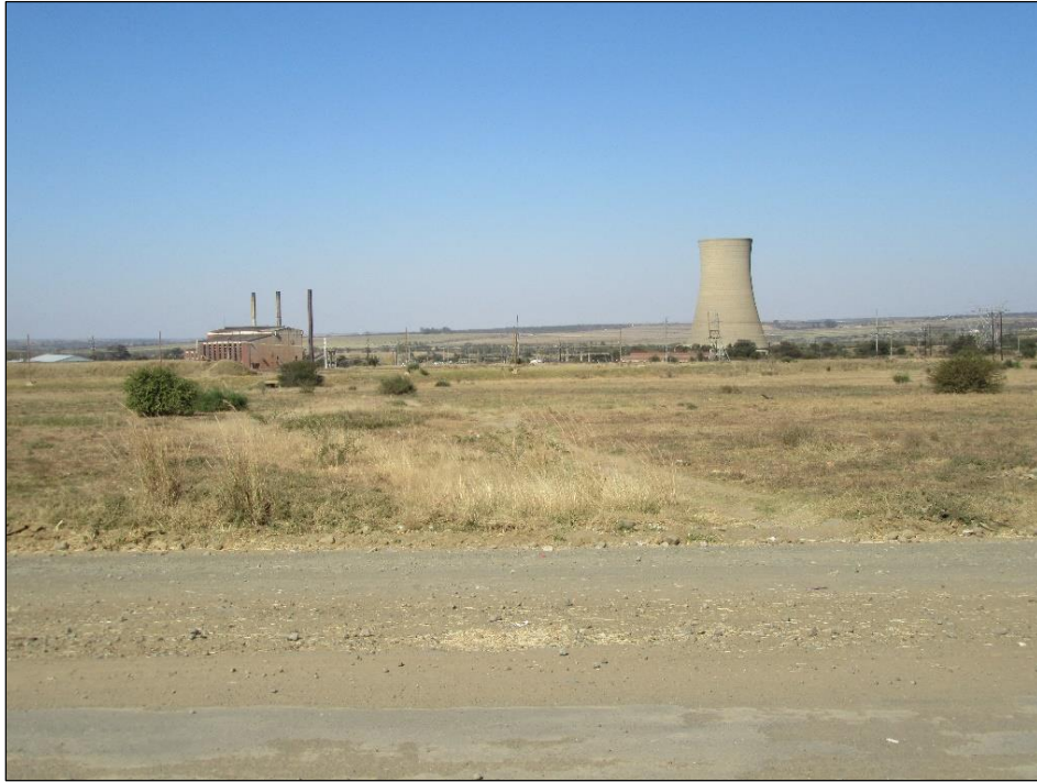
Figure 6: The Old Kroonstad Power Station is a historical landmark located in Industria east of Brent Park.
