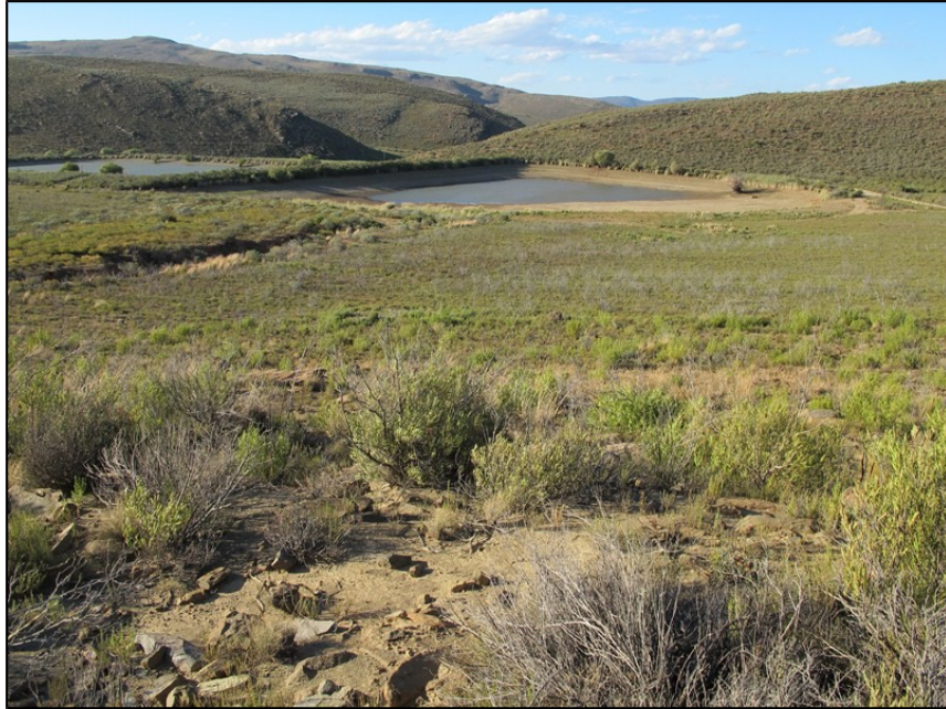
Figure 3: View across the affected area towards the dam in the north. The donga is visible on the left of the photo.
