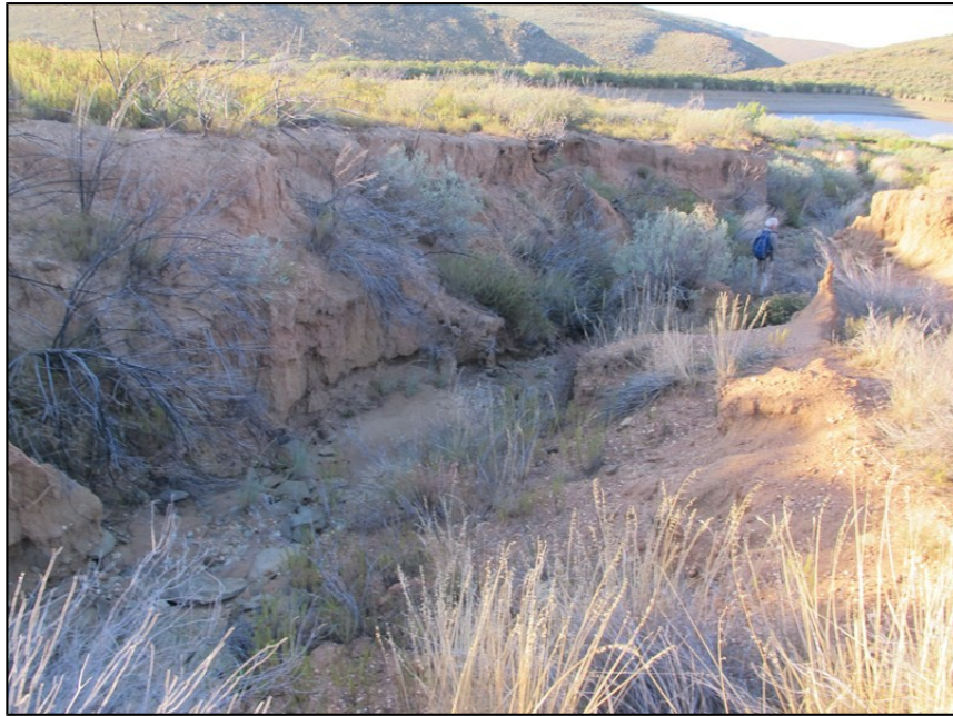
Figure 5: View northwards along the donga to the west of the affected area of pit 25. Slabs of weathered Bokkeveld shale are visible in the bottom of the donga.
