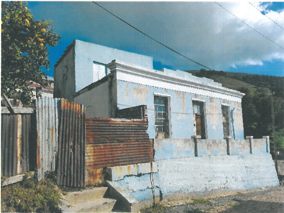
Almonda Street façade
