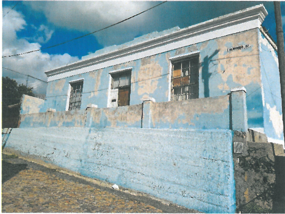
Almonda Street façade
