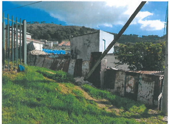
Rear boundary corrugated iron fence
