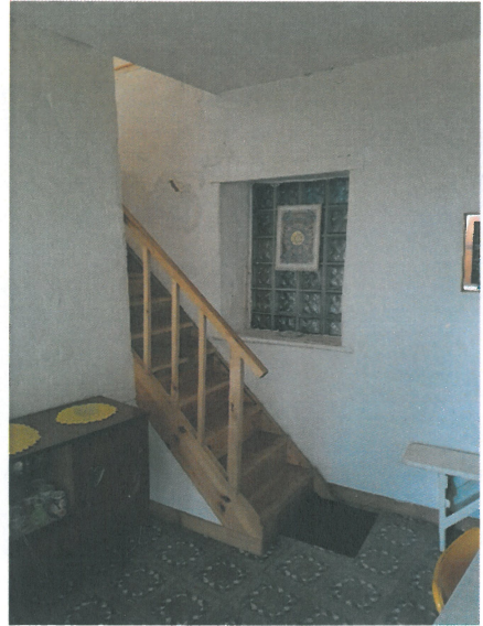
Stair to first floor
