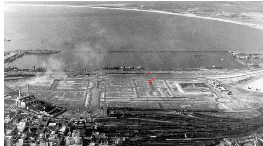
Figure 24: The application of the road network and spatial plan at its purest 1952-1953, prior to later amendments: This shows the Monumental Ceremonial approach (arrowed, through the FGA site) and the Monumental Commercial approach or the Grand Boulevard (Heerengracht/Adderley Street). The Monumental Approach is not yet developed except for the outline of the road framework
