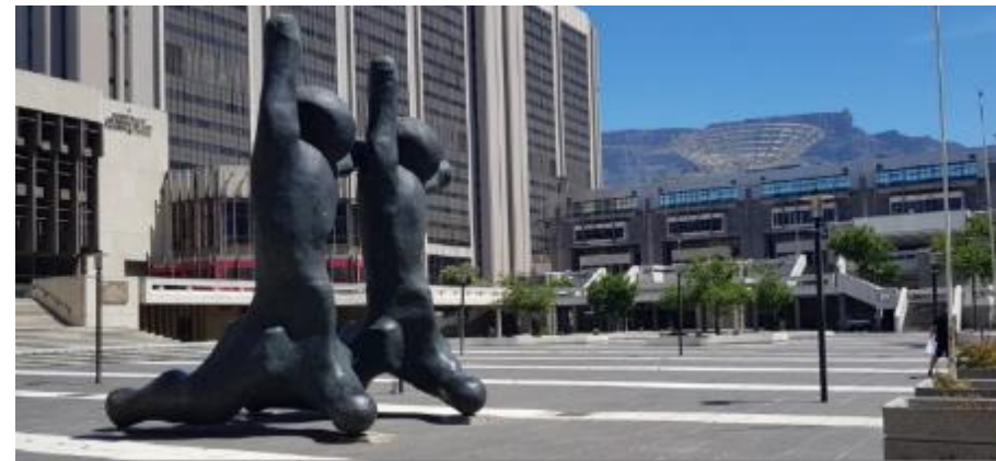
Figure 11: Artscape Plaza with the Civic Centre, it's podium and concourse linking to the Artscape Plaza in the background (@Plan)
