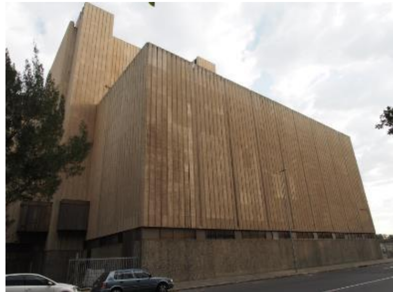
8.4.6 Exterior views- rear and side facades (UDS 2018-20)
