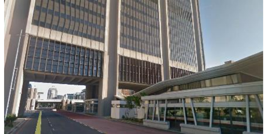
Figure 18: Herzog Boulevard, entering the City from the east, the Civic Centre dominating the entry views and Artscape, right of picture, entirely obscured by the My Citi infrastructure. (Google Earth image).
