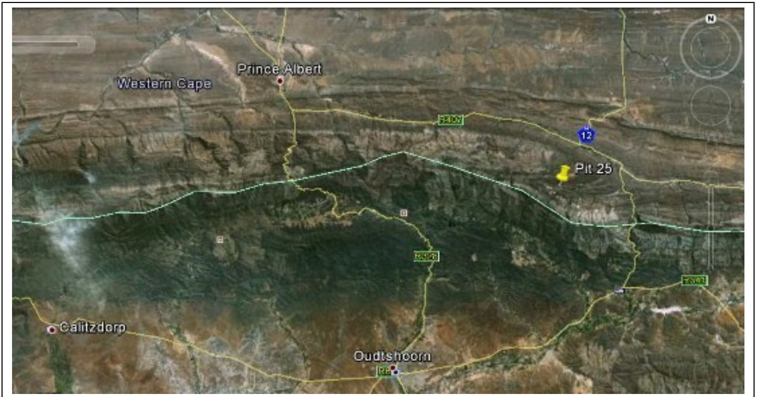
Figure 4: Aerial view of proposed borrow pit location (Tusenius, March 2012)
