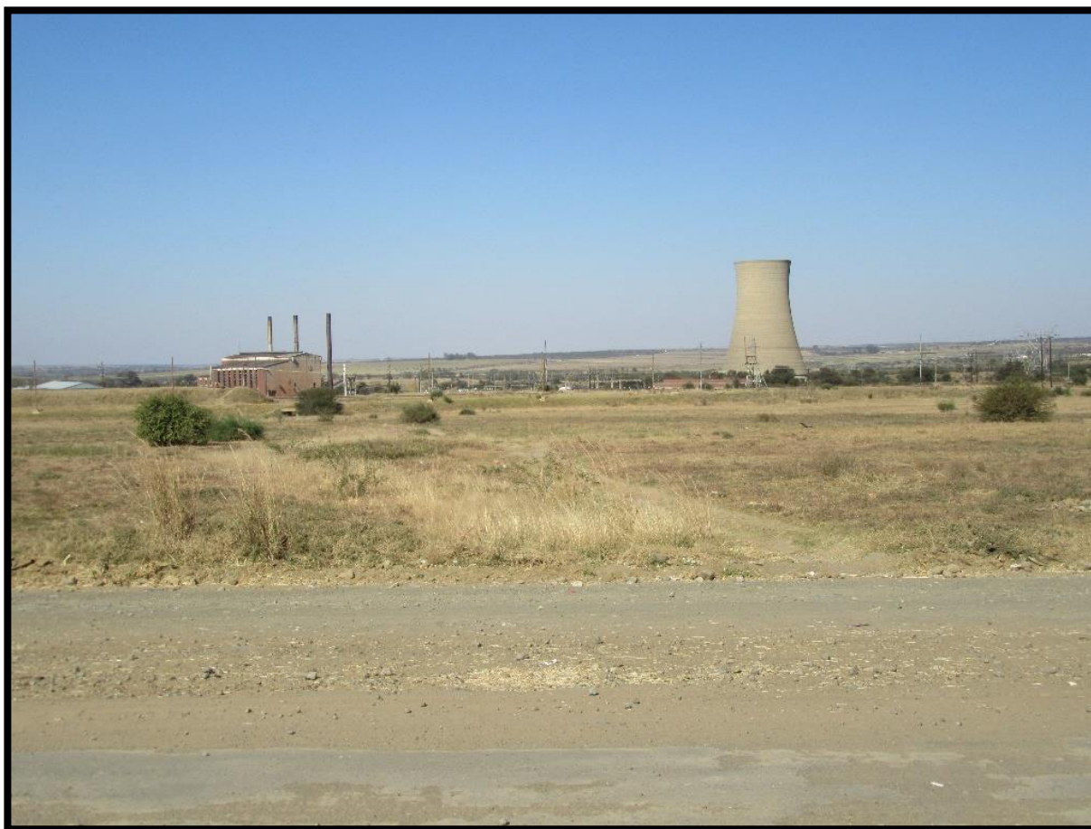
Figure 6: The Old Kroonstad Power Station is a historical landmark located in Industrial east of Brent Park.
