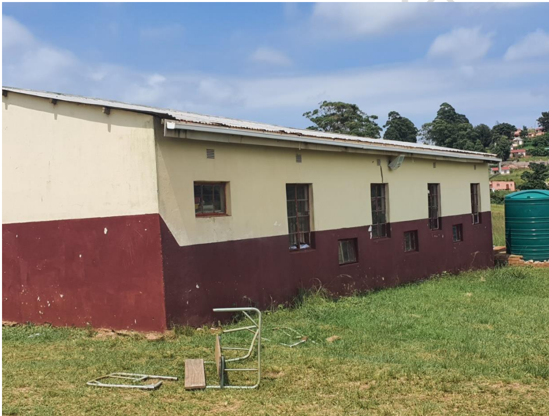
Figure 10; Existing classrooms block
