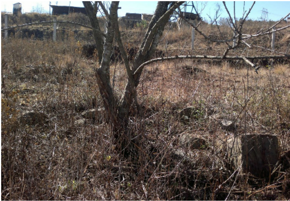
Figure 6: Remains of foundation / wall of structure
