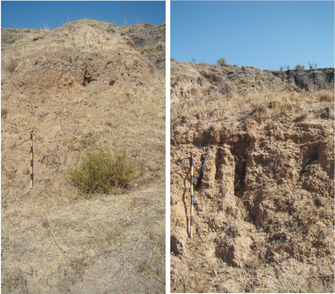
Figure 10. The channel alluvium along the Sand River are mostly made up of grey and red to yellow sandy clays reaching a thickness of up to 5.0 m in places.
