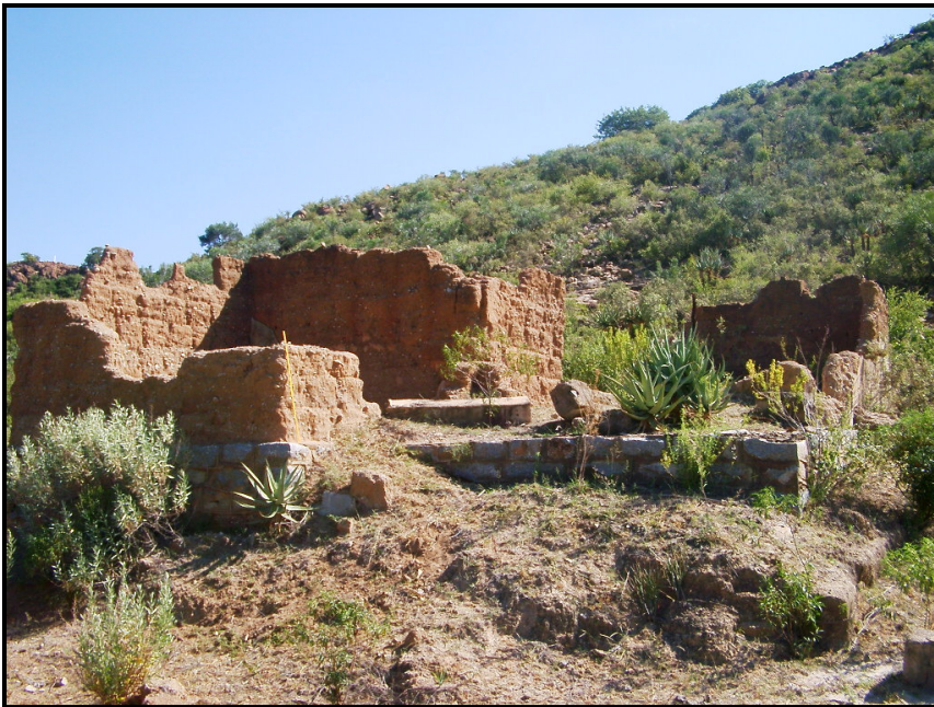
Figure 16. Construction of the houses - stone foundation, with adobe walls (Unit 2).
