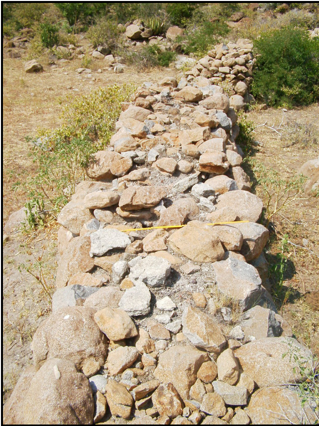
Figure 21. Construction technique of the freestanding stone walls: two rows of boulders filled in with smaller pieces of stone and rubble.
