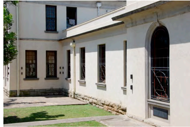
External burglar bars over windows
