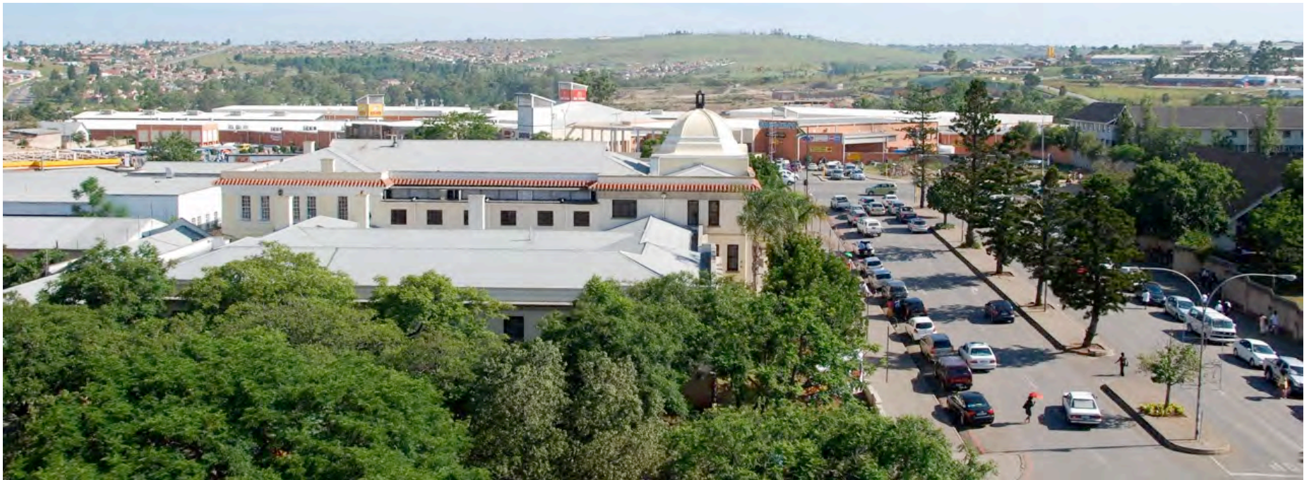
Bhunga Building from the North, within context of Mthatha, July 2010. Owen Road on right hand side 6
