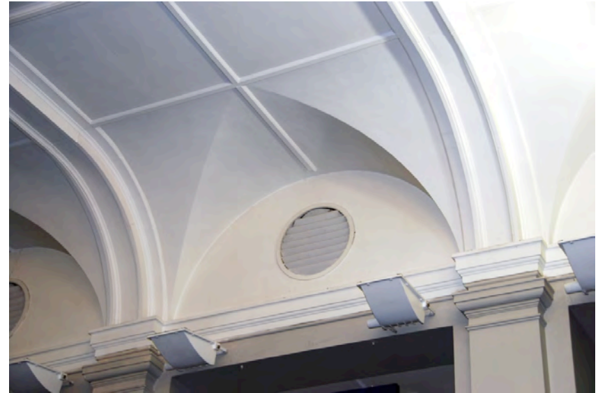
Vaulted ceiling in Council Chamber
