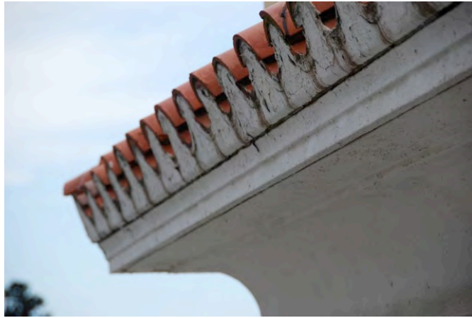
Deep overhanging moulded cornice
