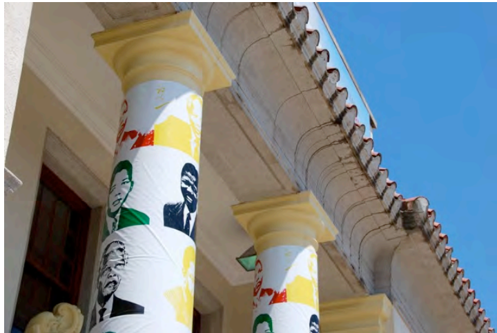
Columns and column capitals to entrance portico
