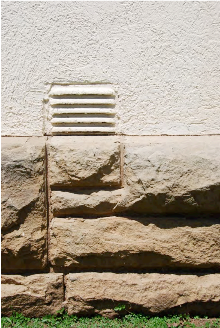
Louvred airbrick, later textured wall coating and stone plinth
