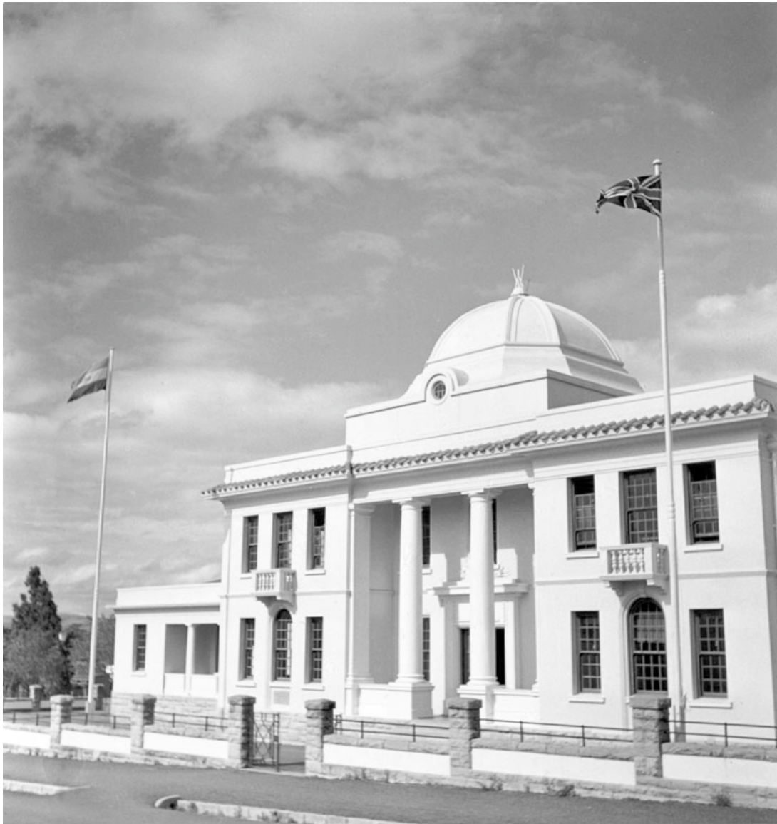
The General Council Building at Umtata; West Elevation onto Owen Street, 1947. Photographed by Larrabee, C S, 1914 - 2000. Smithsonian Institution, National Museum of African Art, Eliot Elisofon Photographic Archive, EEPA_1998_061358 General Council Building
