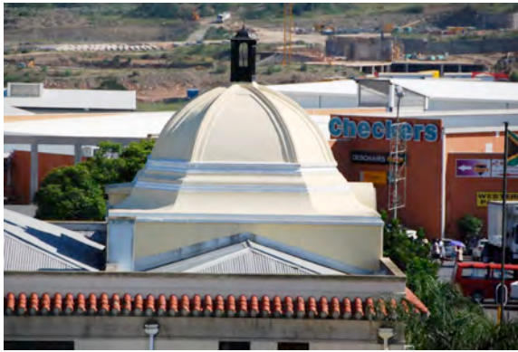
Plastered concrete dome and timber finial
