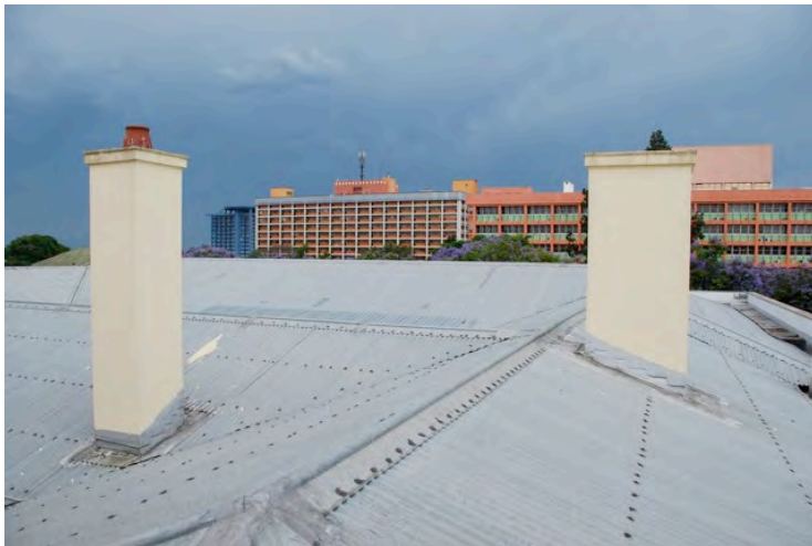
Hipped corrugated iron roof with plastered chimney stacks
