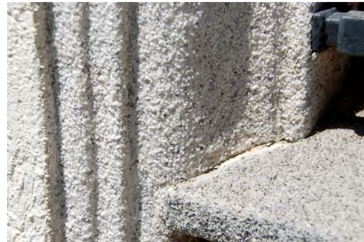
Details of moulding to window surround obscured by textured plaster
