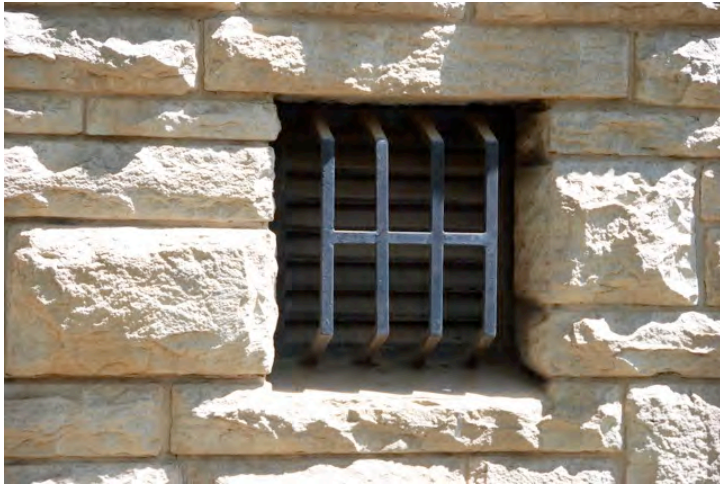
Louvred ventilator in hammer dressed sandstone plinth
