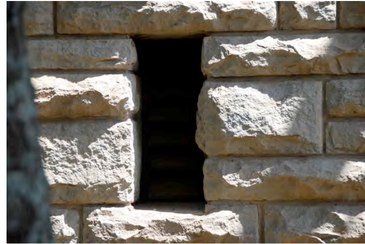
Rectangular opening in hammer dressed sandstone plinth
