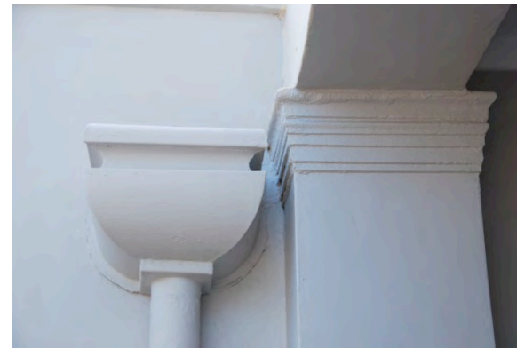
Moulded sheet metal rainwater head and column capital
