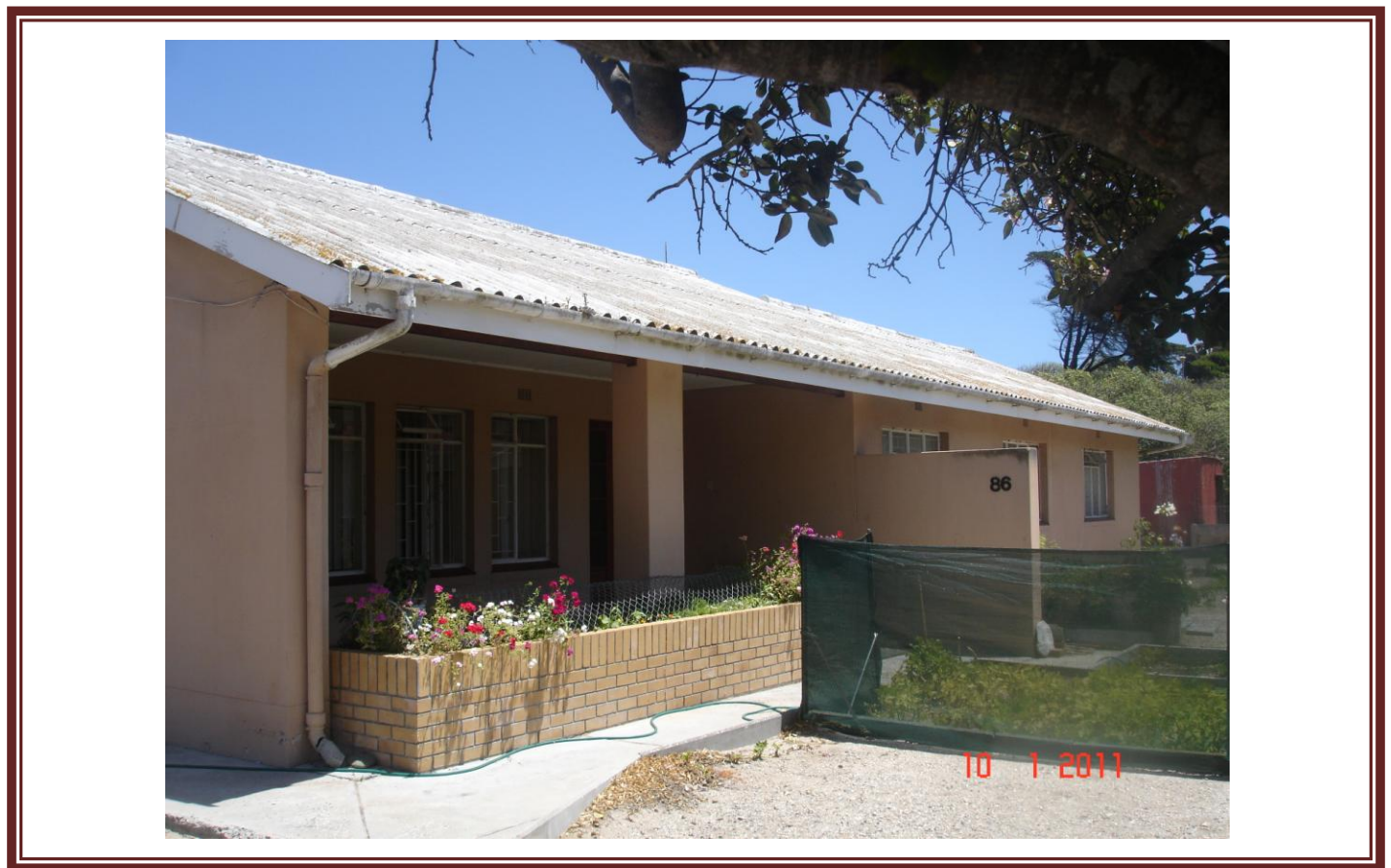
Fig.6.2. North face main entrance.
