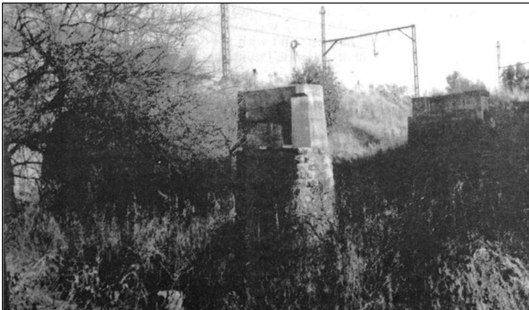
Figure 18: Remaining sandstone abutments of the Moreleta Spruit bridge (after De Jongh 1988).
