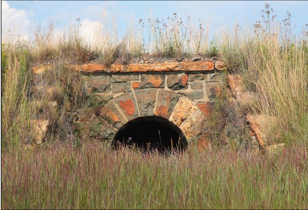
Figure 13: Well preserved stone culvert east of Delfsand Property.
