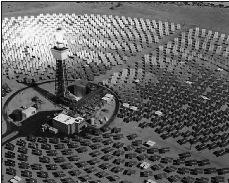
Figure 3 - An example of a power plant using central receiver technology. This is a 10MW demonstration plant that was built in the United States – image courtesy NREL.
