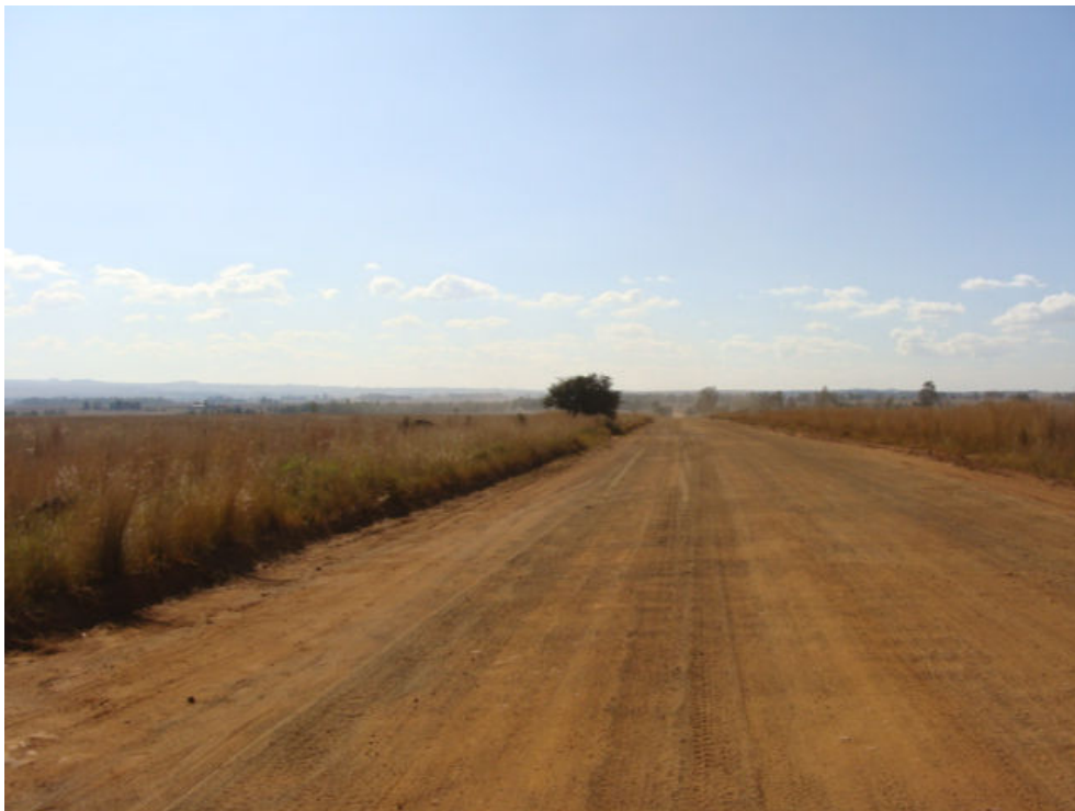
Figure 9 View of western section of section 2.
