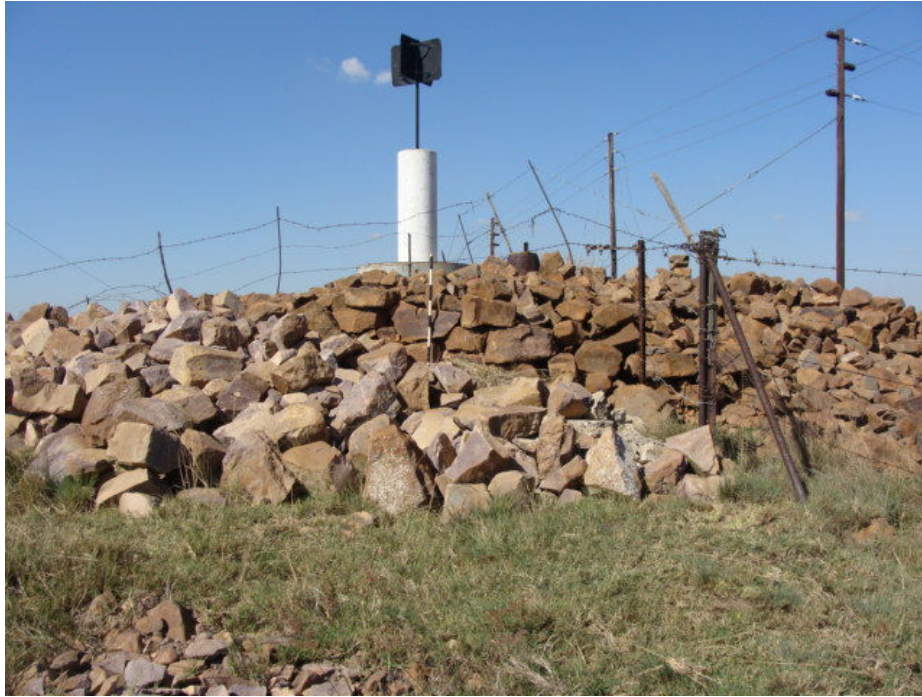
Figure 16 The basis of the blockhouse. The lighter colored stones in the front were placed there much later.
