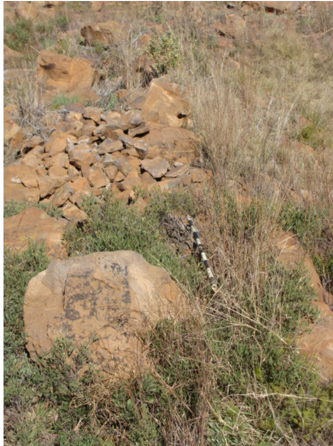
Figure 14 Stone enclosure at the blockhouse consisting of two parallel walls filled in with stones, very typical of military structures.
