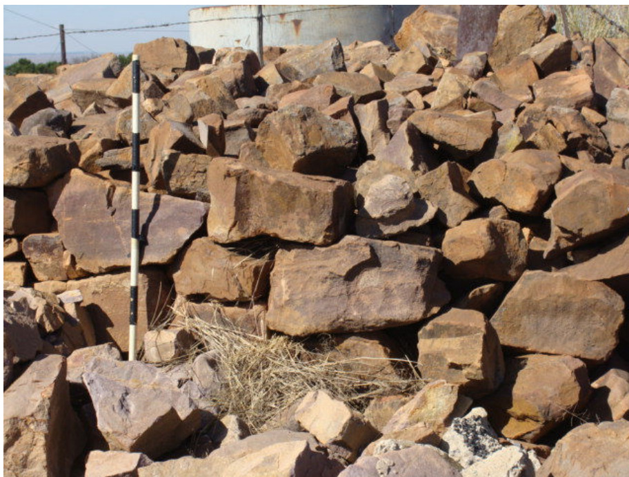
Figure 15 Close up of a wall that forms part of the basis of the blockhouse.
