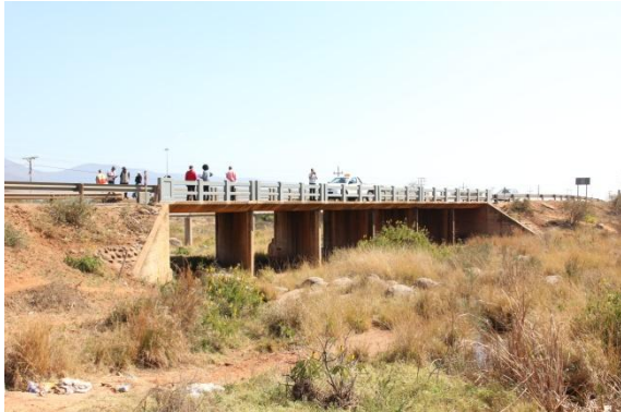
Showing the embankments on both sides of the bridge.
