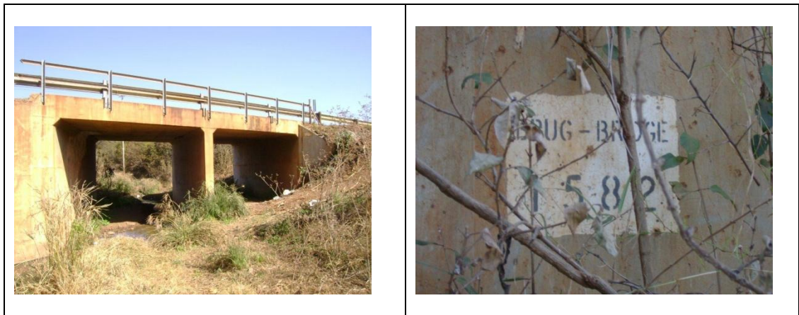
Fig. 5. Side-view of the bridge and its identification number.
