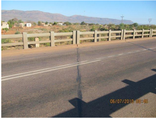
Bridge deck seen from the top
