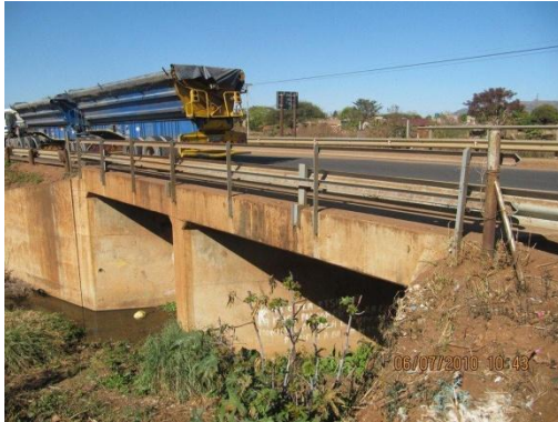
Railing on eastern side of bridge
