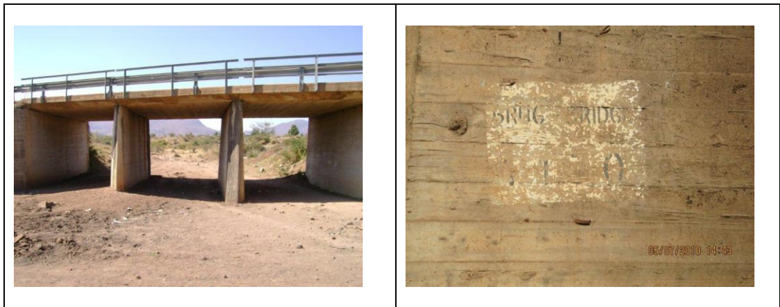
Fig. 11. Side-view of the bridge and its identification number.
