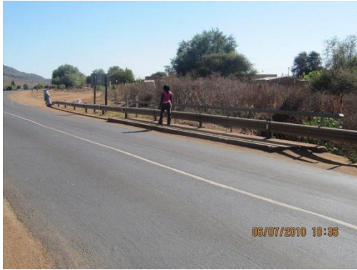
Bridge deck seen from the top
