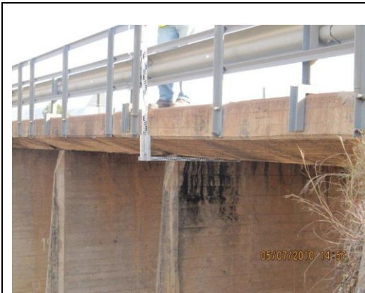
Railing on eastern side of bridge
