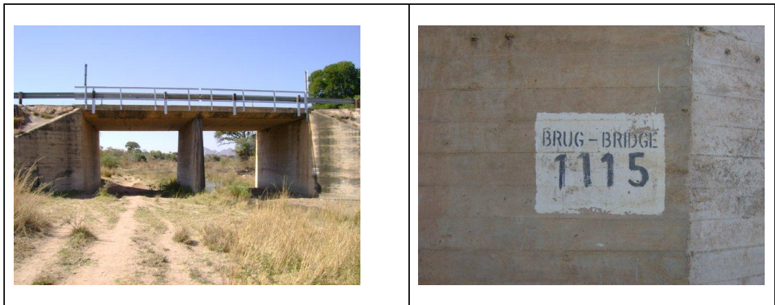
Fig. 14. Side view and identification number of the bridge.
