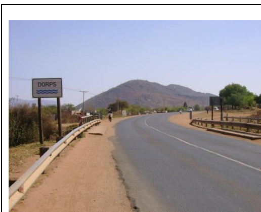
Approach road, travelling north
