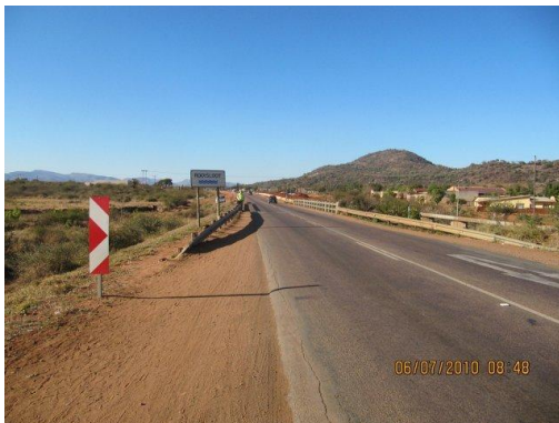
Approach road, travelling north
