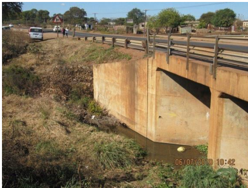
Showing the south-eastern embankment
