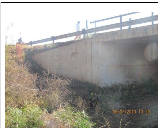
Abutment wall, north-eastern side
