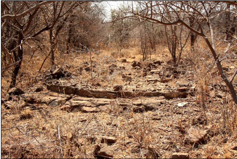
Figure 5-12: Cement and brick foundation structure of a dam and house at Site HP01.
