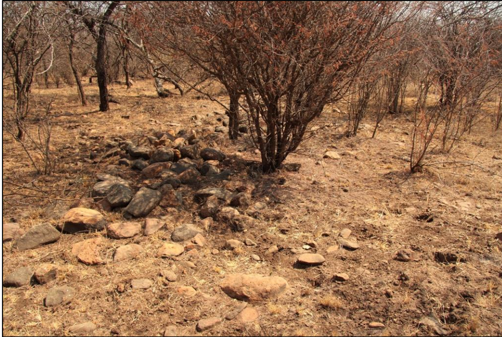
Figure 5-7: Collapsed stone wall section at Site IA02
