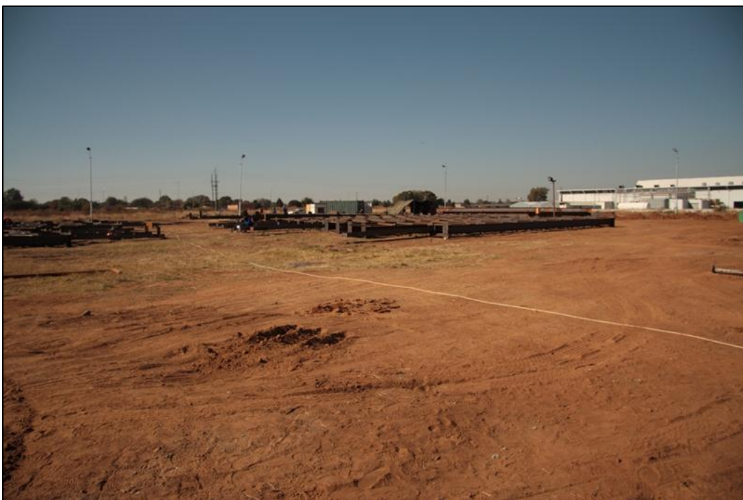
Figure 6: Infrastructure construction and material at the Babelegi steel recycling facility.
