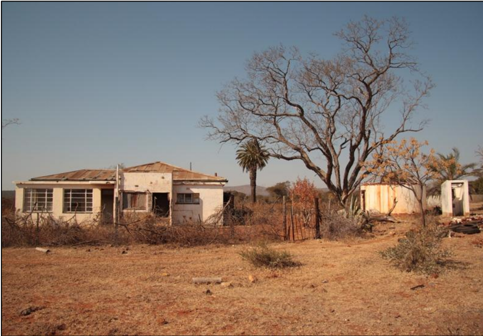
Figure 5-24: Various structures at the old Ruigedraai homestead (Site HP03).
